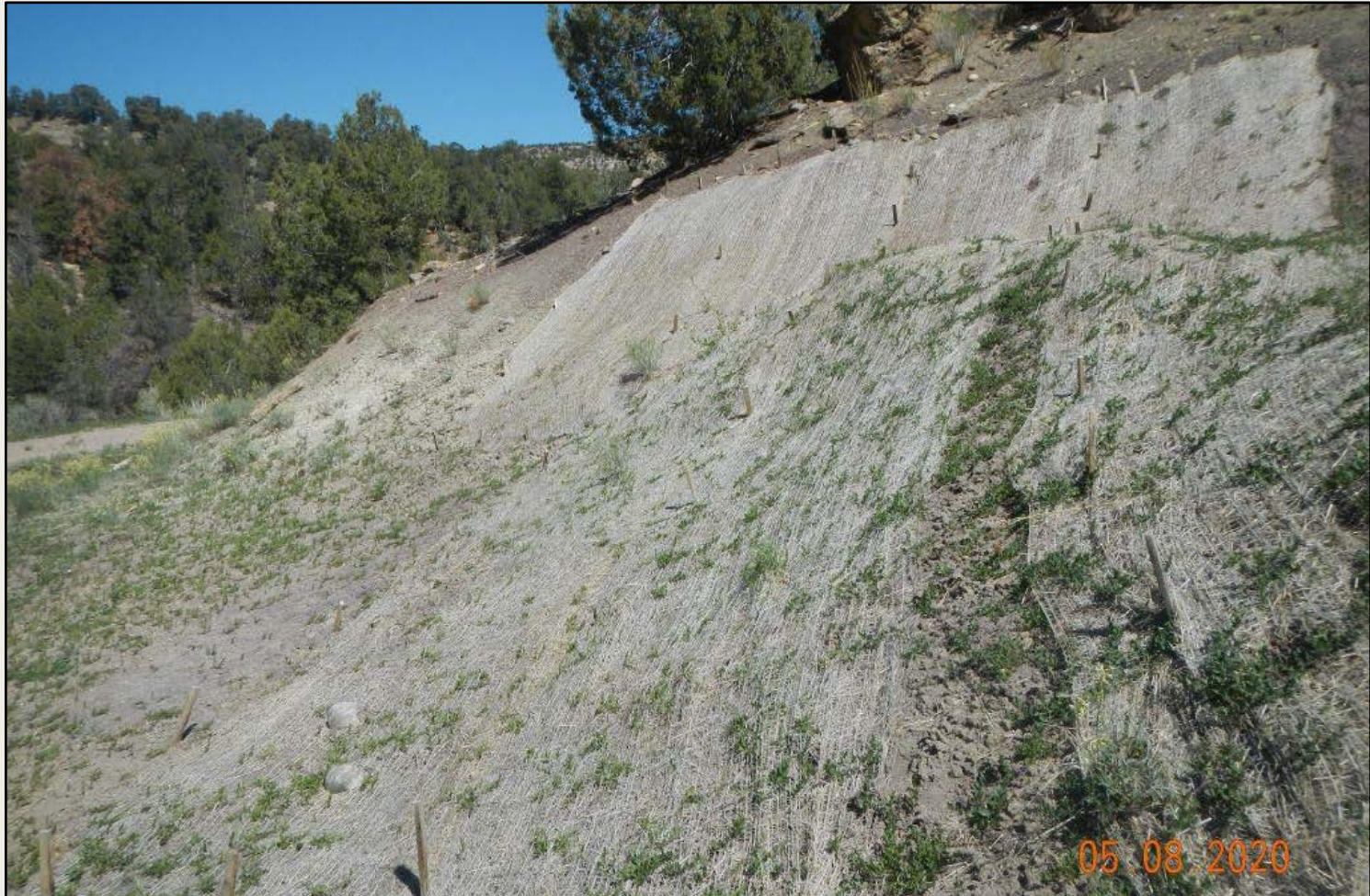
Photo 3. View of erosion control blanket placed on northeastern cut-slope.
