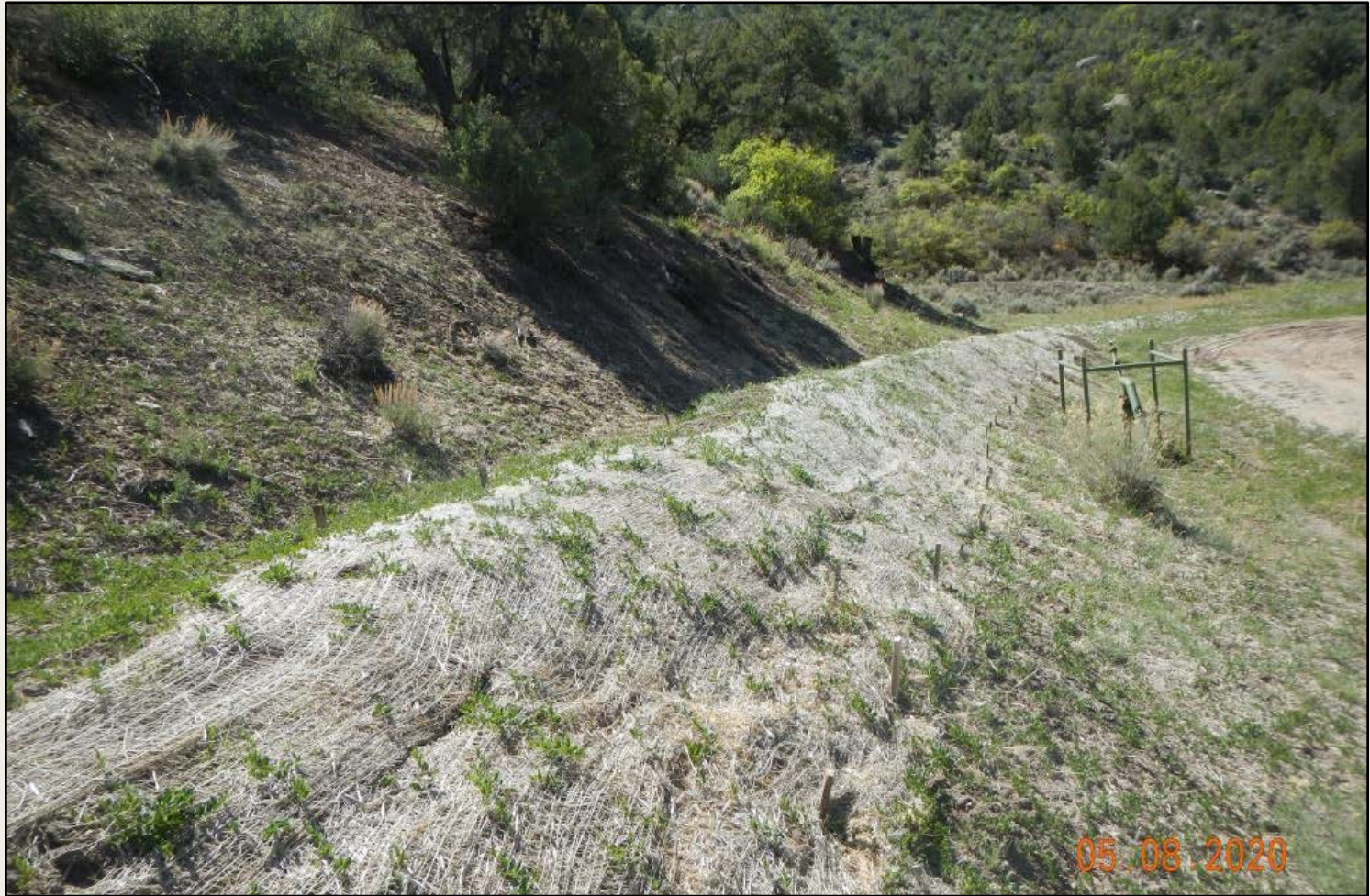
Photo 2. View of the eastern project area from the northeastern corner facing southward. Erosion control blanket appears to be functioning. Cut-slopes are seeded/straw-mulched in response to 2018 reclamation inspection.
