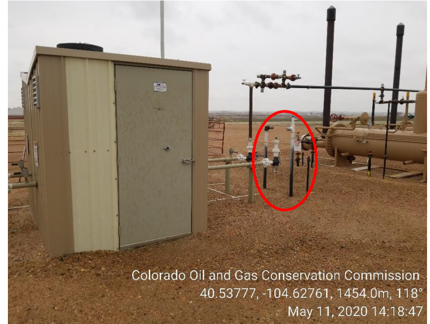
Photo 14: Unused risers, disconnected gas meter
