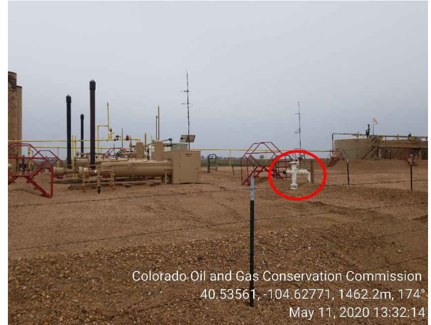
Photo 4: Equipment, gas meter removed; riser remains
