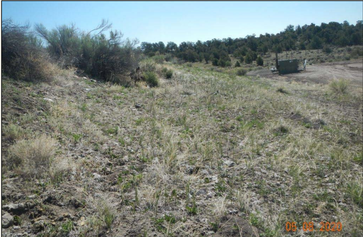
Photo 5. View of the central fill slope between two well pads from the southwestern corner facing eastward. Fill slope was seeded in 2018, some grasses such as smooth brome becoming established here. Hydromulch still visible. Poor germination observed on portions of the slope.
