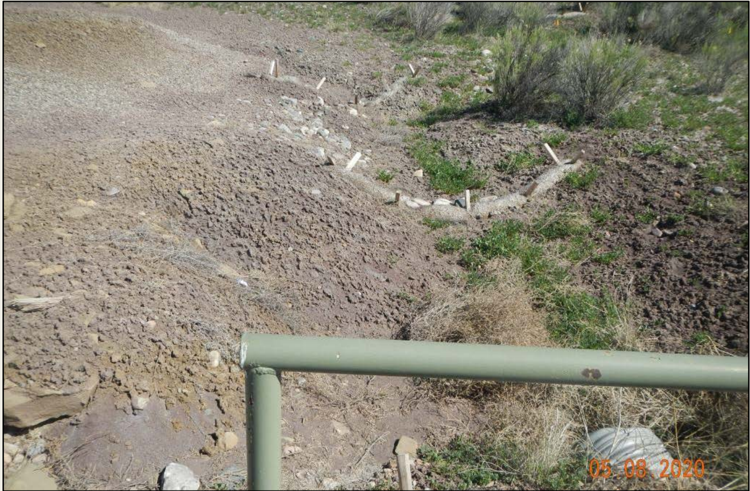
Photo 10. View of culvert inlet at the entrance to the southern well pad. Bare soils are not stabilized, wattles and cobble are full of sediment.
