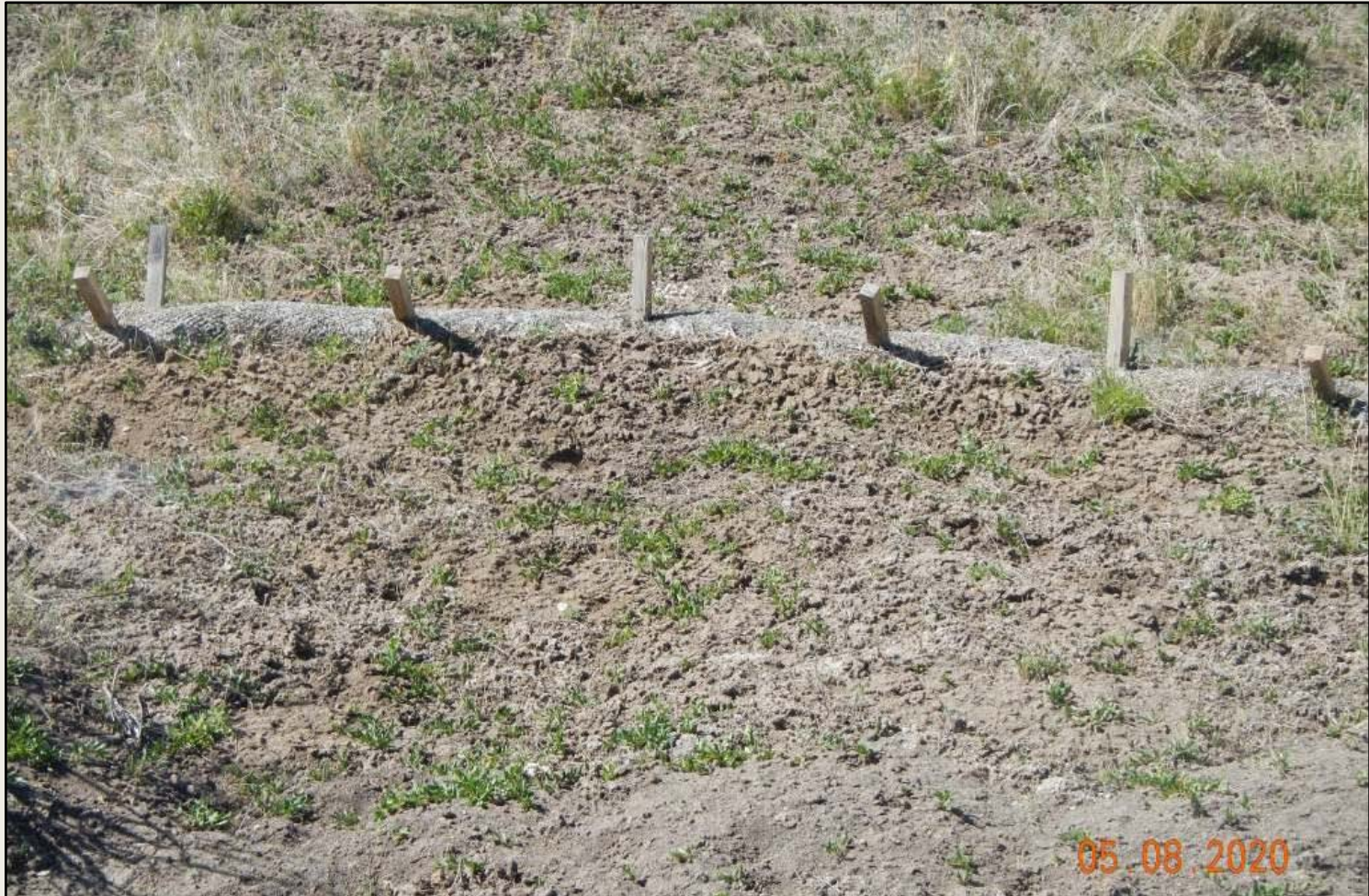
Photo 8. View of another wattle in the southern fill slope that is full of sediment.
