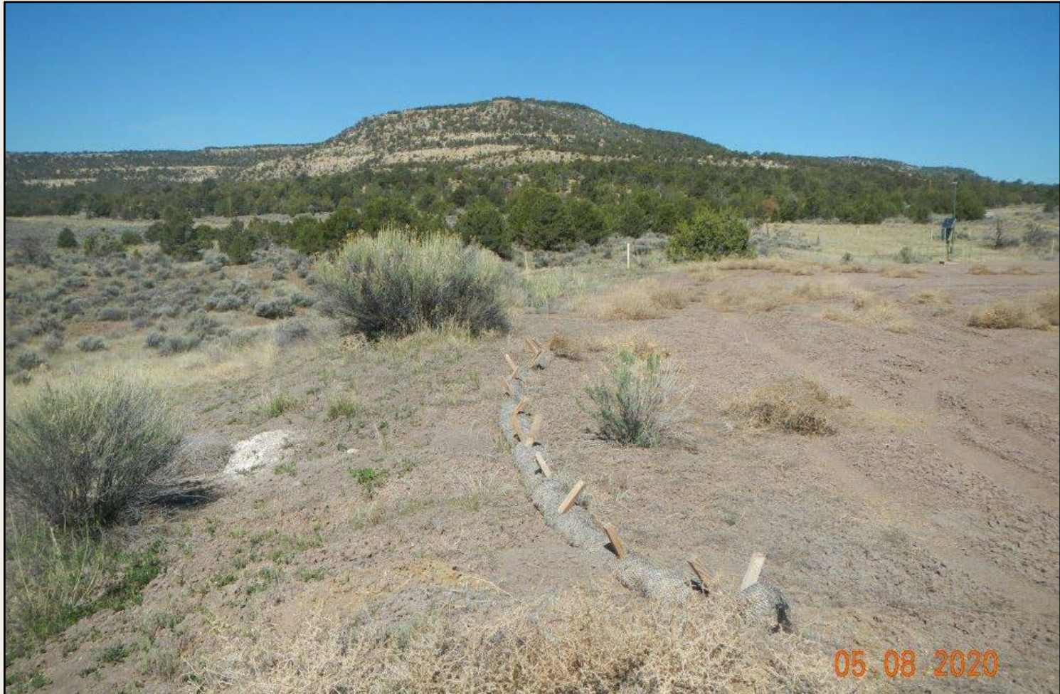
Photo 7. View of the southern fill slope facing westward. Wattle is full of sediment and needs maintenance.
