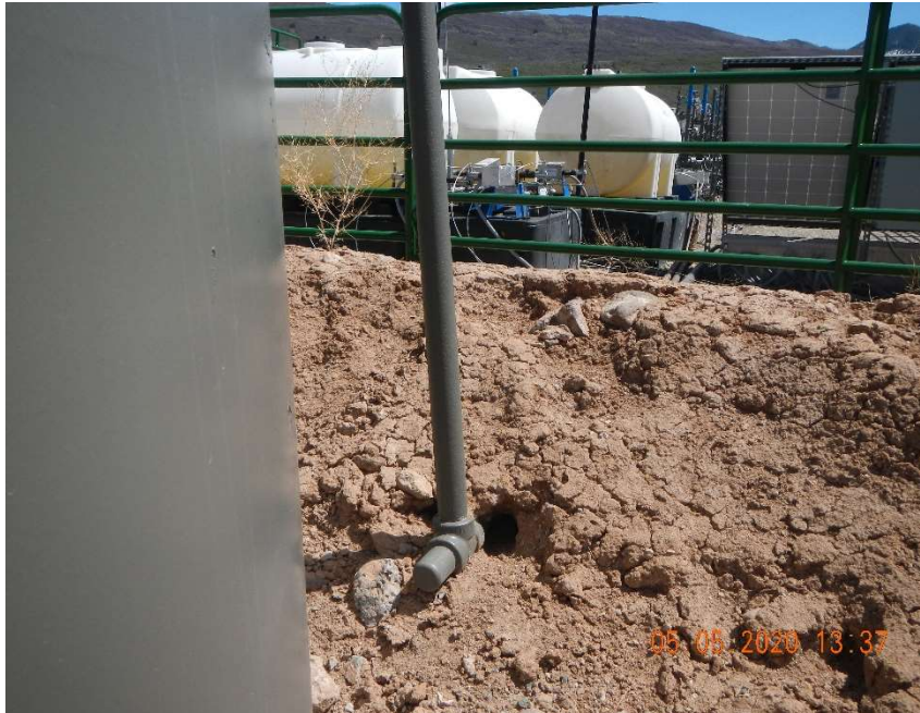
5/5/2020 2-inch flowline penetrating the earthen secondary containment
