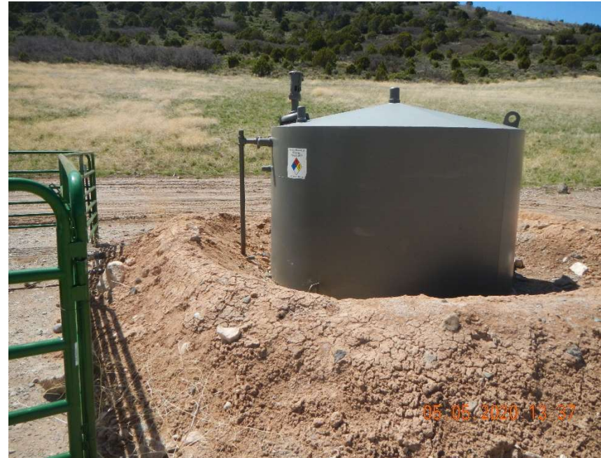
5/5/2020 80 bbl produced water steel AST with earthen secondary containment
