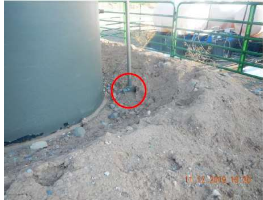
11/12/2019 2-inch flowline penetrating the earthen secondary containment
