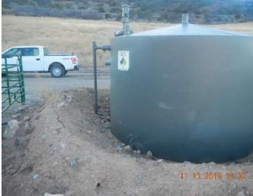
11/12/2019 80 bbl produced water steel AST with earthen secondary containment
