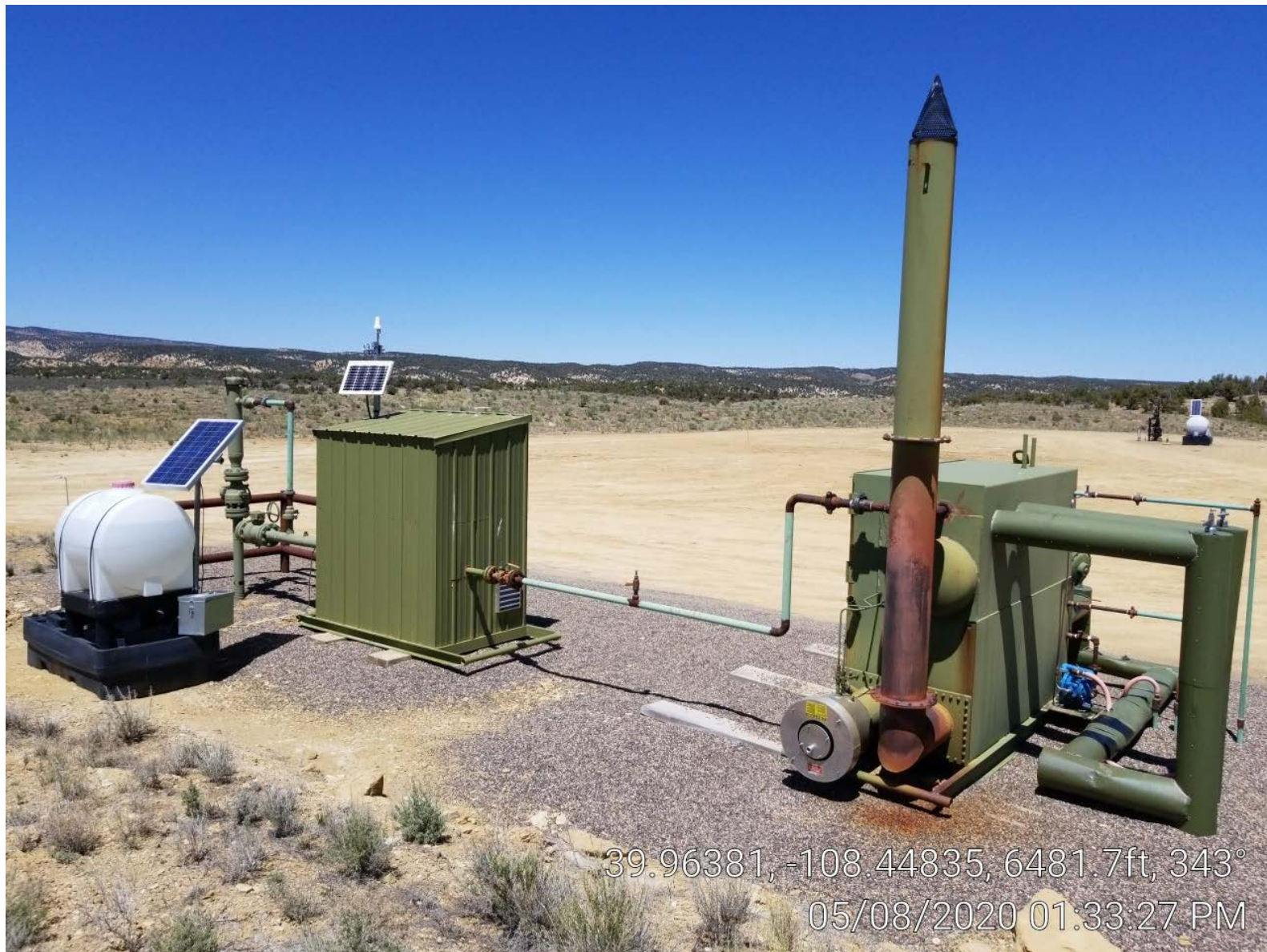
Photo 4. Meter building & separator.
