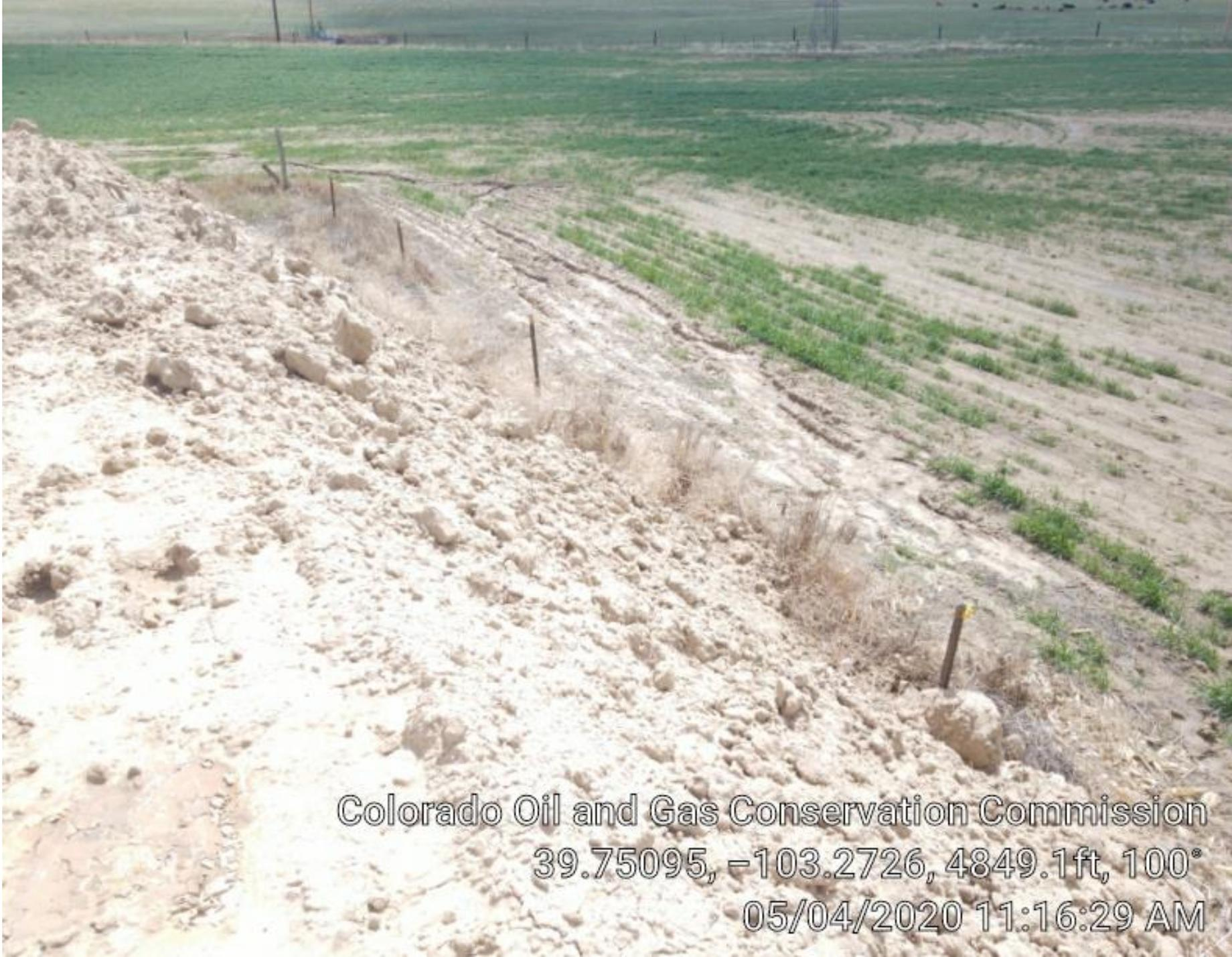
Area on south side of produced water pit berms where berm breached and spilled into field.
