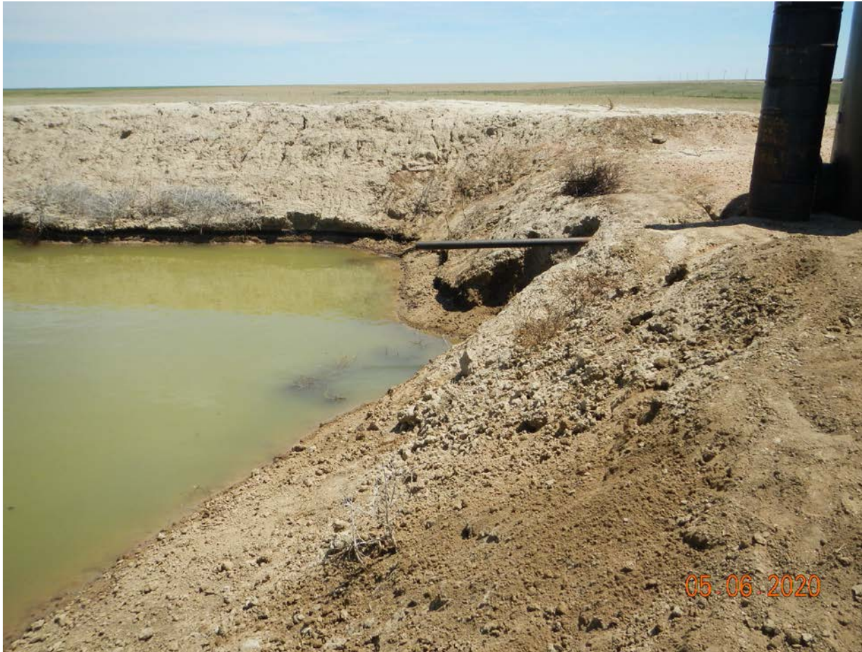
Photo # 4 – Oil skim tank outfall to produced water pit ID 117639
