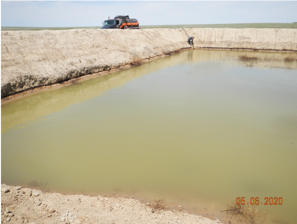
Photo # 6 – Produced water pit ID 117639 view NNW. Vacuum truck on site removing crude oil from surface of pit. Wind from SSE.
