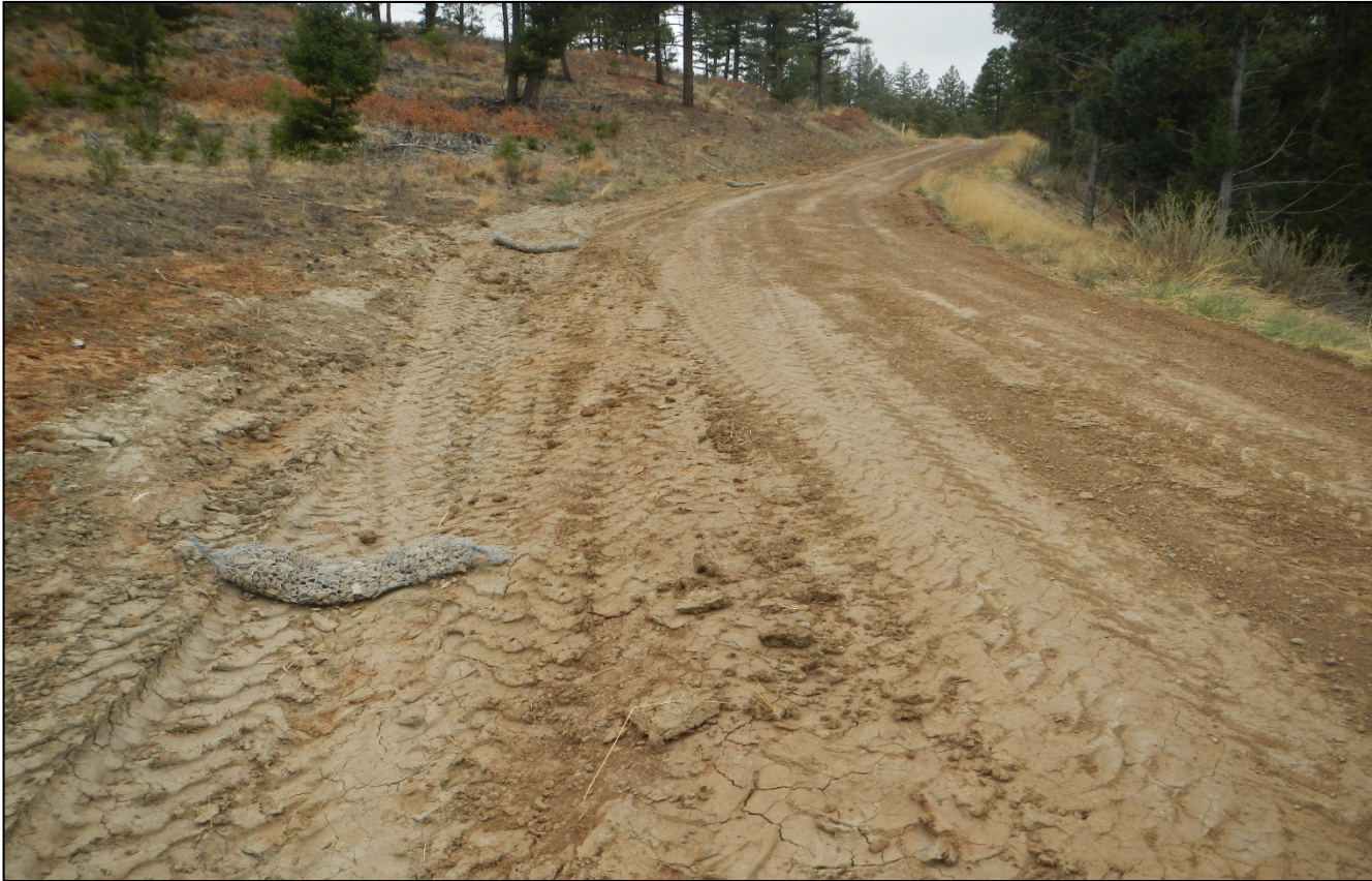
Photo 1. Facing southwest along the access road. The road has been graded and culverts are maintained. Rock sock check dams have been installed along the side. The check dams will need to be monitored to ensure stormwater does not flow around the sides.
