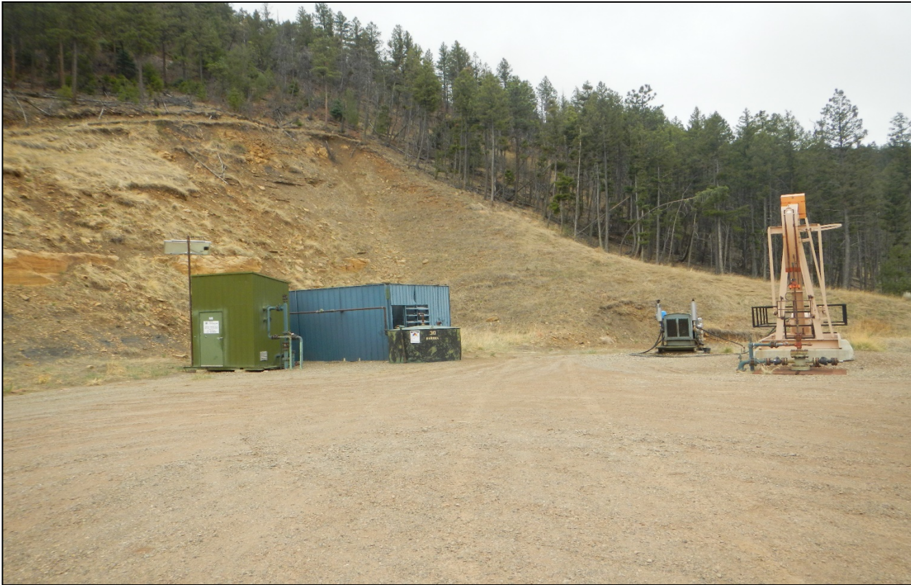
Photo 1. Facing southwest toward the location.
