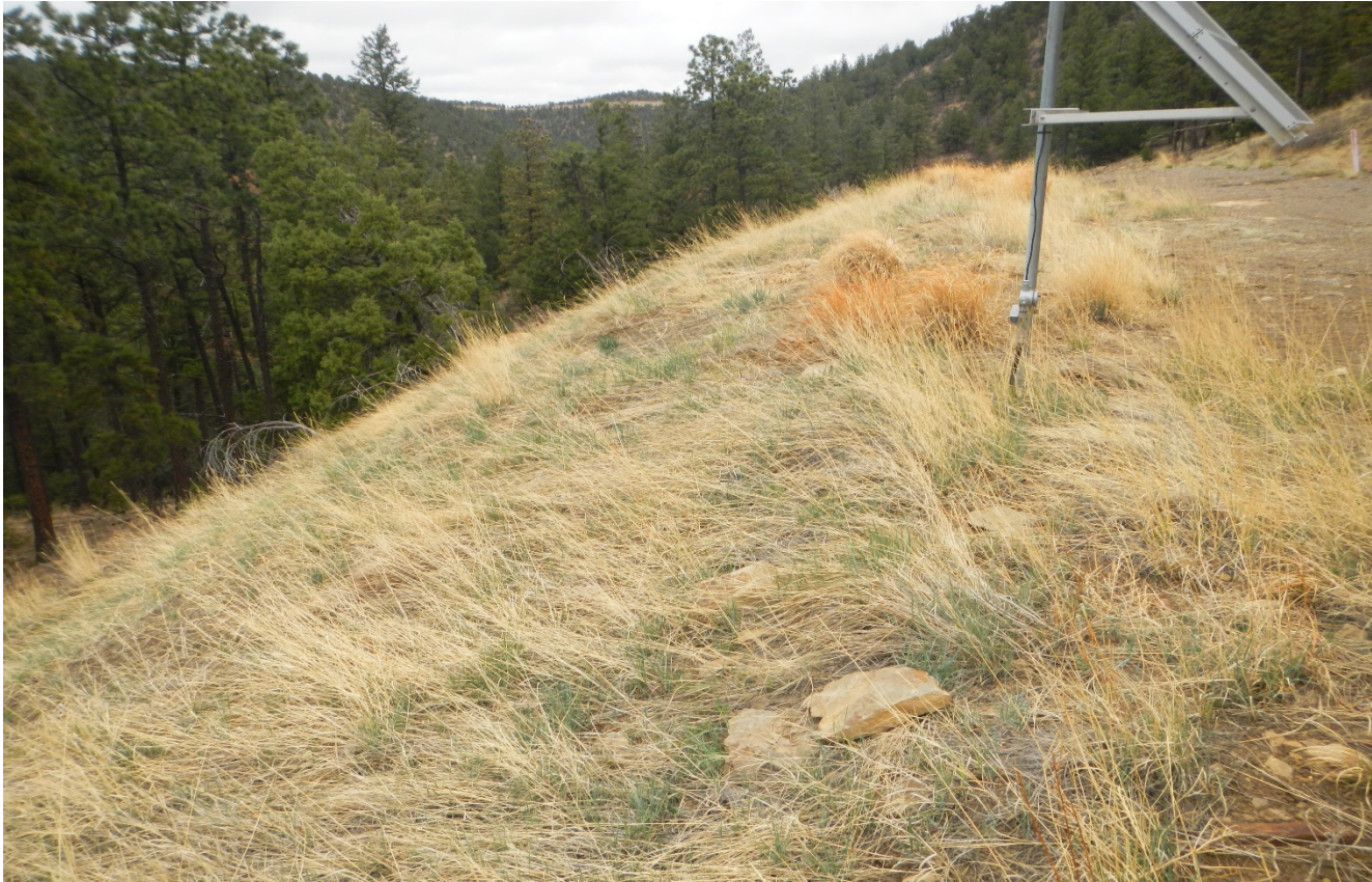
Photo 4. Facing toward the fill slope which is stabilized with vegetation.
