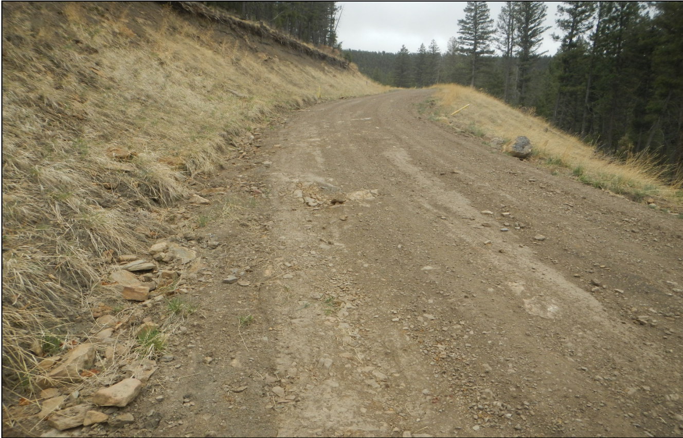
Photo 2. Facing west along the access road. The road has been graded and large rock moved off the road.
