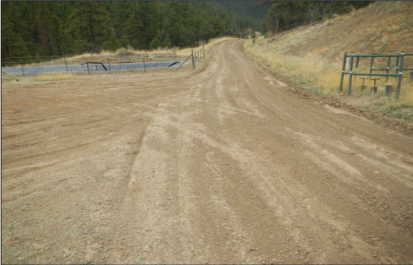
Photo 1. Facing southwest along the access road near the GE 31-04 site. The road has been graded and maintained.
