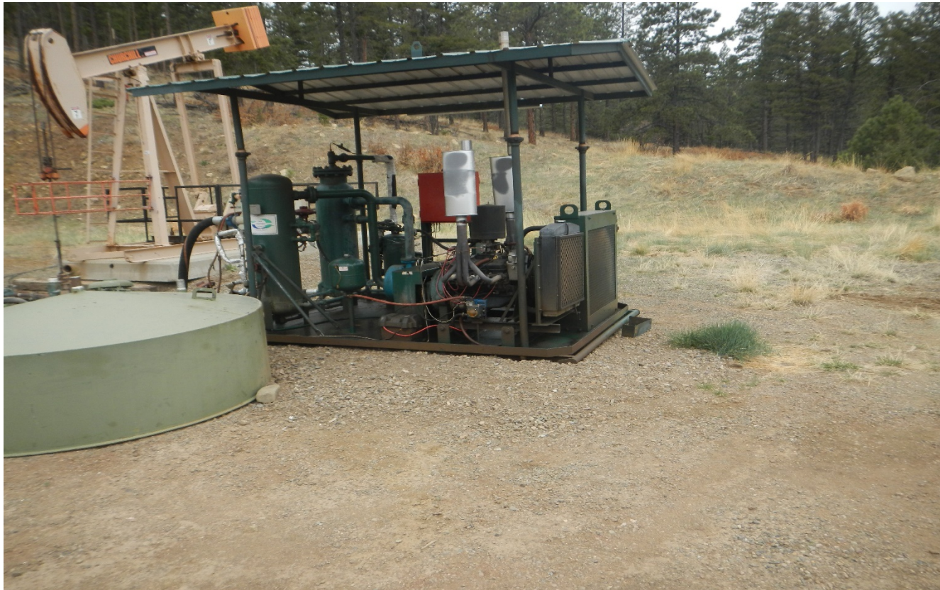
Photo 5. The oil in the engine skid has been cleaned up.
