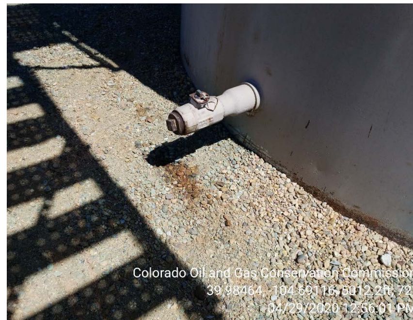
Photo 4 – Minor soil staining observed at base of tank
