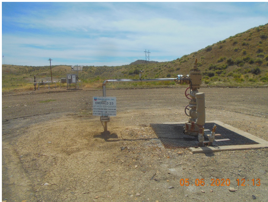
Injection wellhead
