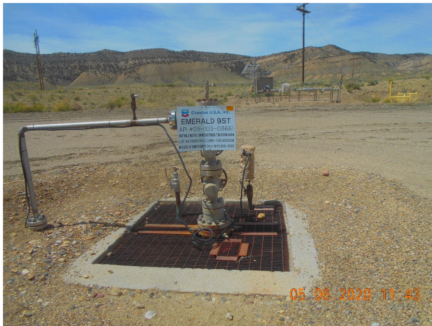
Injection wellhead
