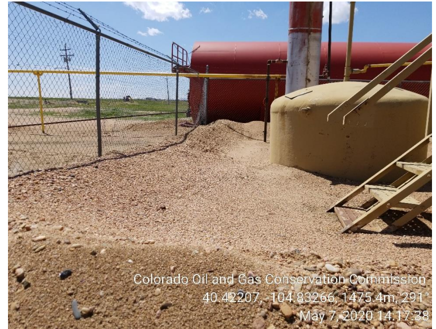
Photo 10: Inadequate berm
