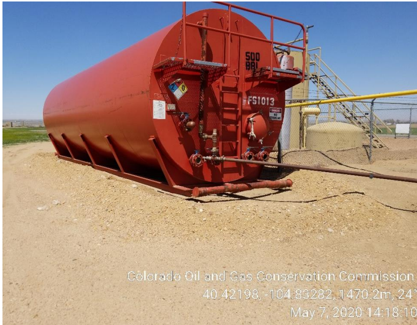
Photo 11: Tank not grounded
