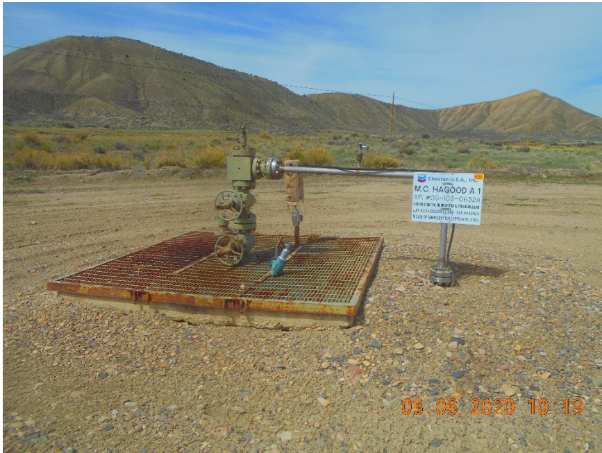
Injection wellhead
