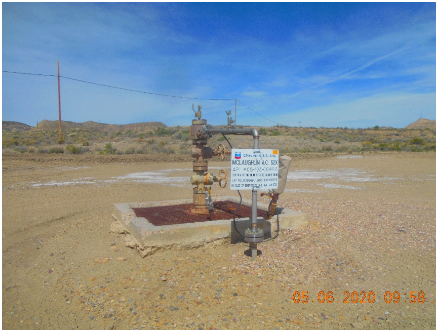
Injection wellhead
