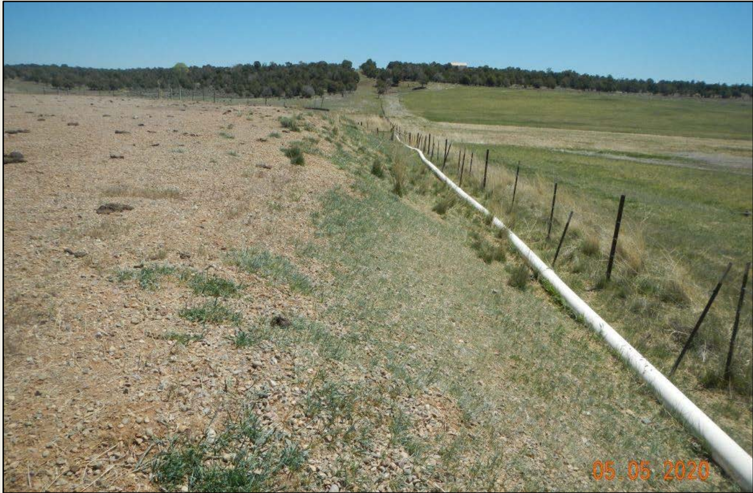
Photo 2. View of the southern fill slope from the southeastern corner facing westward. Revegetation is progressing with western wheatgrass, intermediate wheatgrass, and smooth brome.
