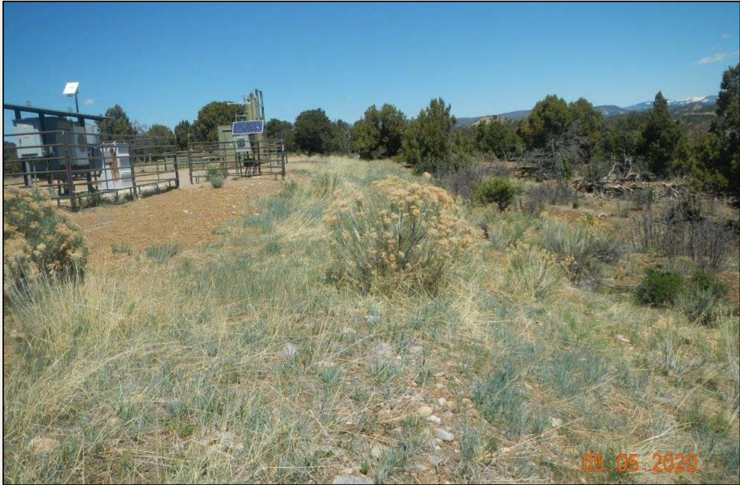
Photo 2. View of the eastern fill slope from the southeastern corner facing northward. Revegetation is progressing largely with western wheatgrass, rubber rabbitbrush, and sand dropseed.
