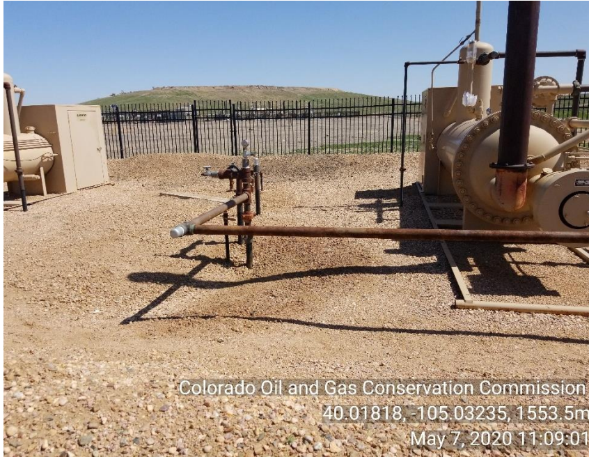
Photo 7 stained soil in separator containment
