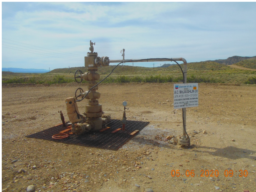
Injection wellhead.
