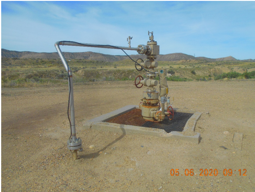
Injection wellhead
