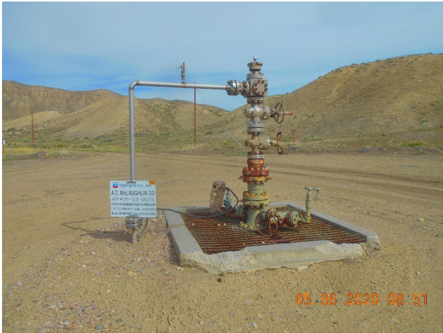
Injection wellhead
