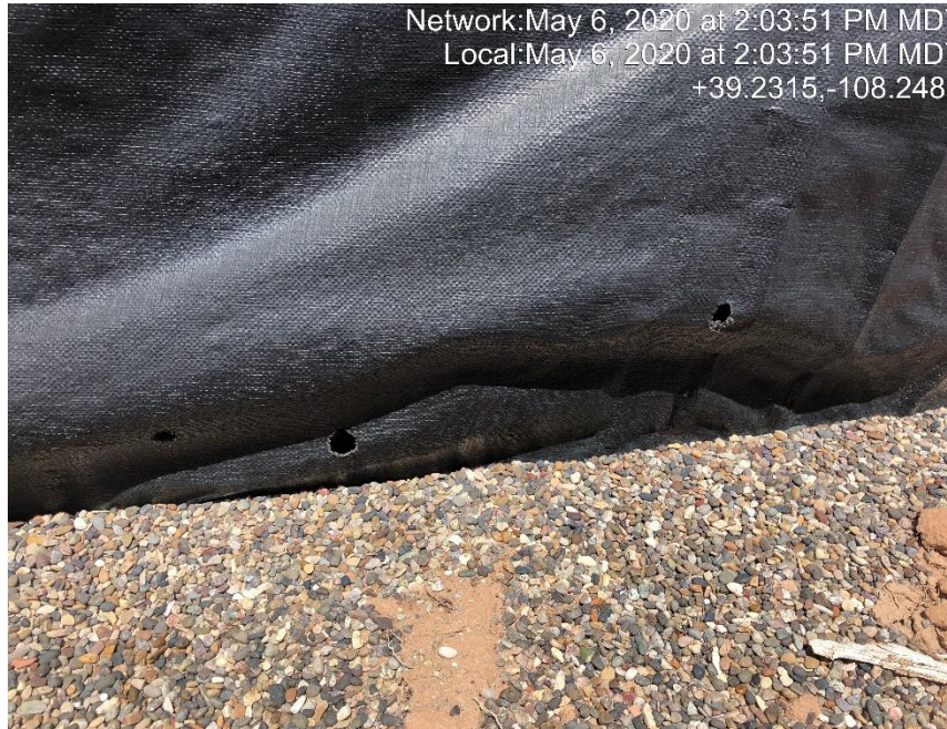
Photo #1134 Multiple holes in tank containment liner.
