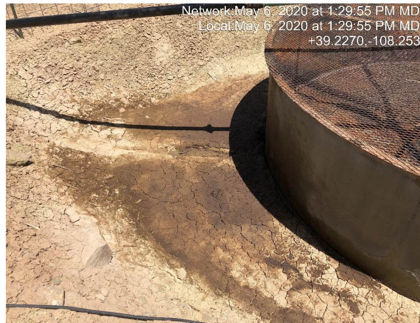
Photo #1131 Stained soil inside tank containment.
