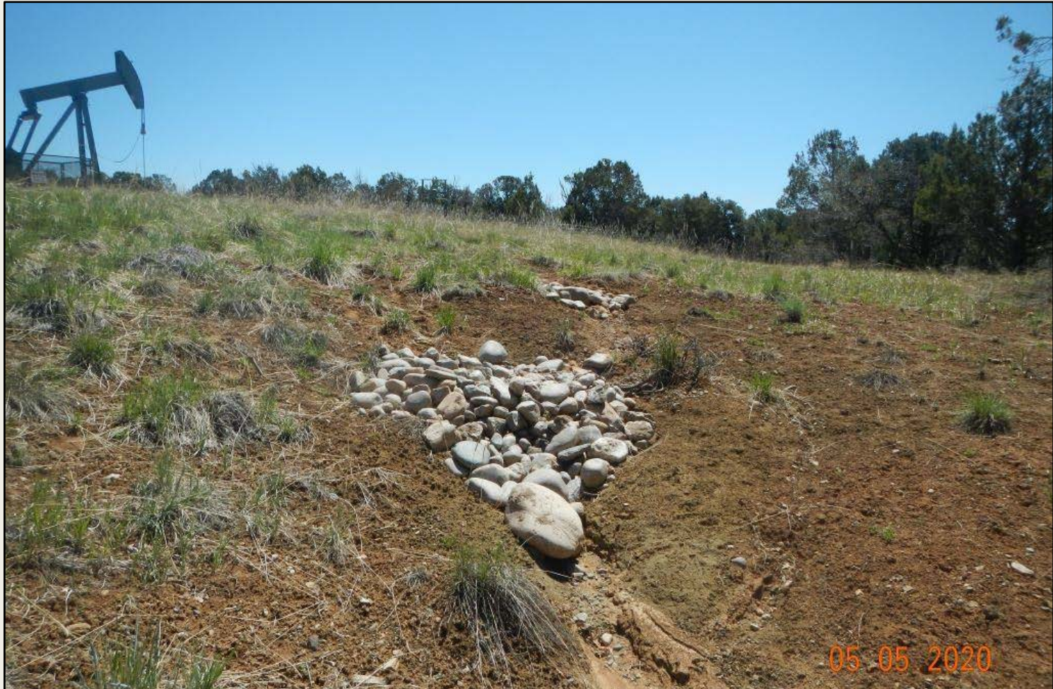
Photo 4. View of cobble bare in the southwestern project area. Erosional scouring and sediment transport continuing between BMPs.
