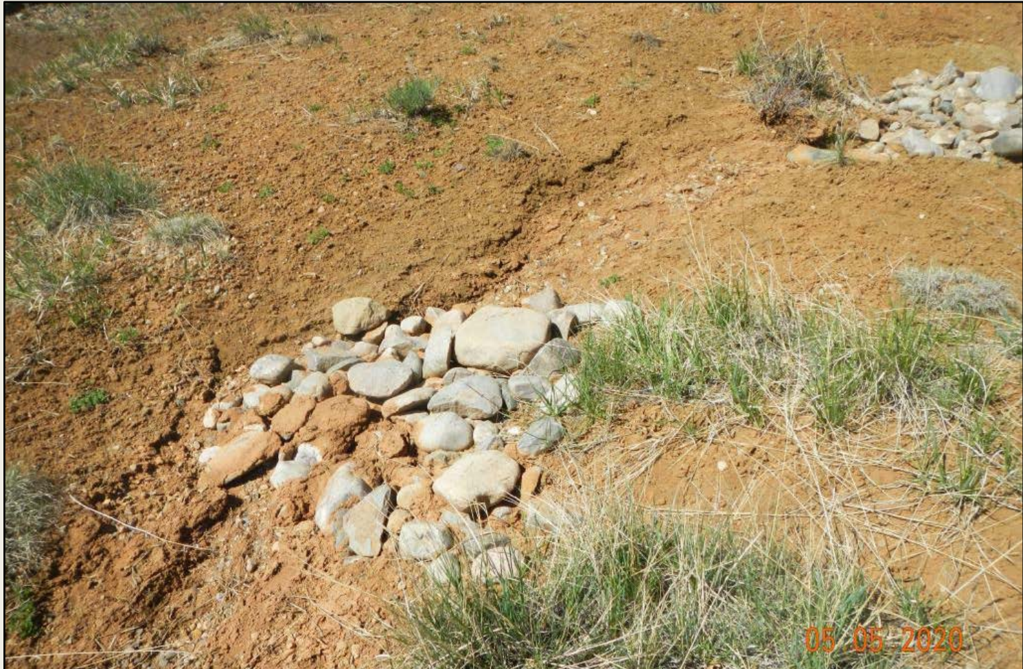
Photo 3. View of cobble placed in southwestern erosional channel. Erosion is continuing around cobble and between cobble bars, as it is not an adequate BMP in this area. Additional BMPs are needed.
