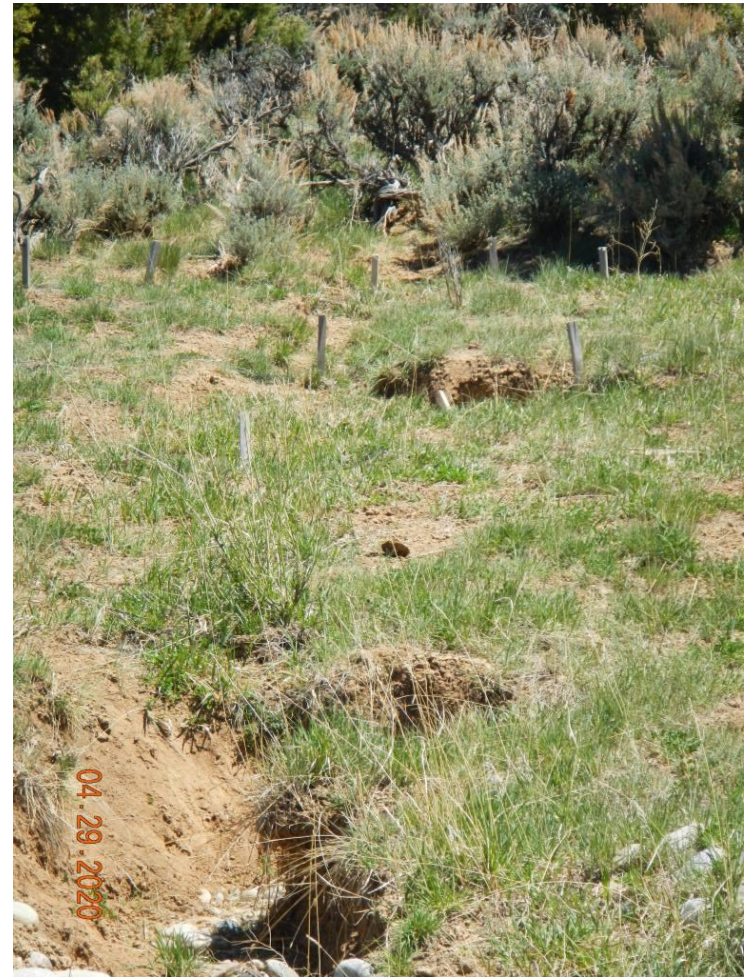
Photo#7: Erosion down gradient of access road culvert.
