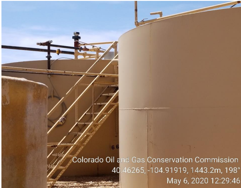
Photo 57: Tanks are not anchored
