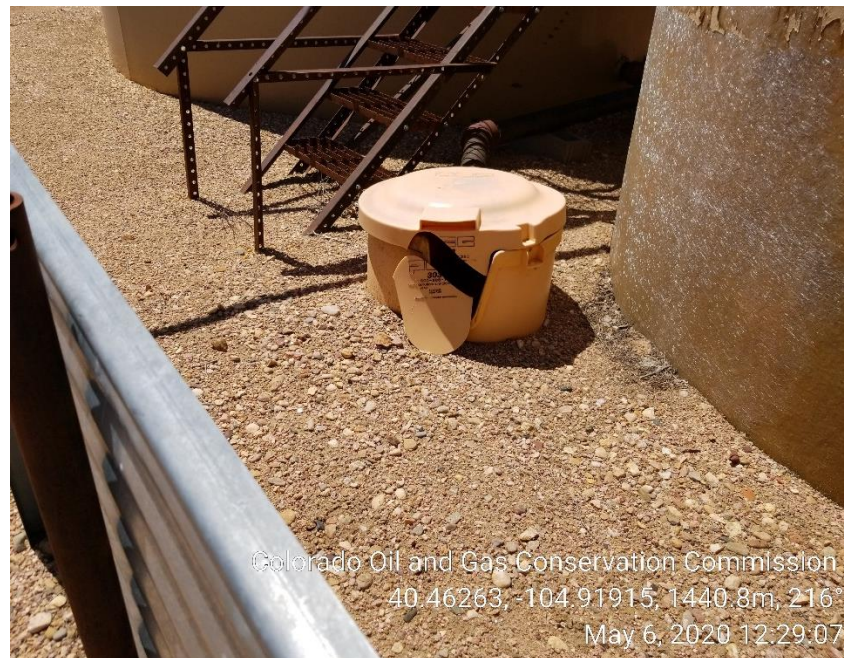
Photo 56: Load out bucket damaged
