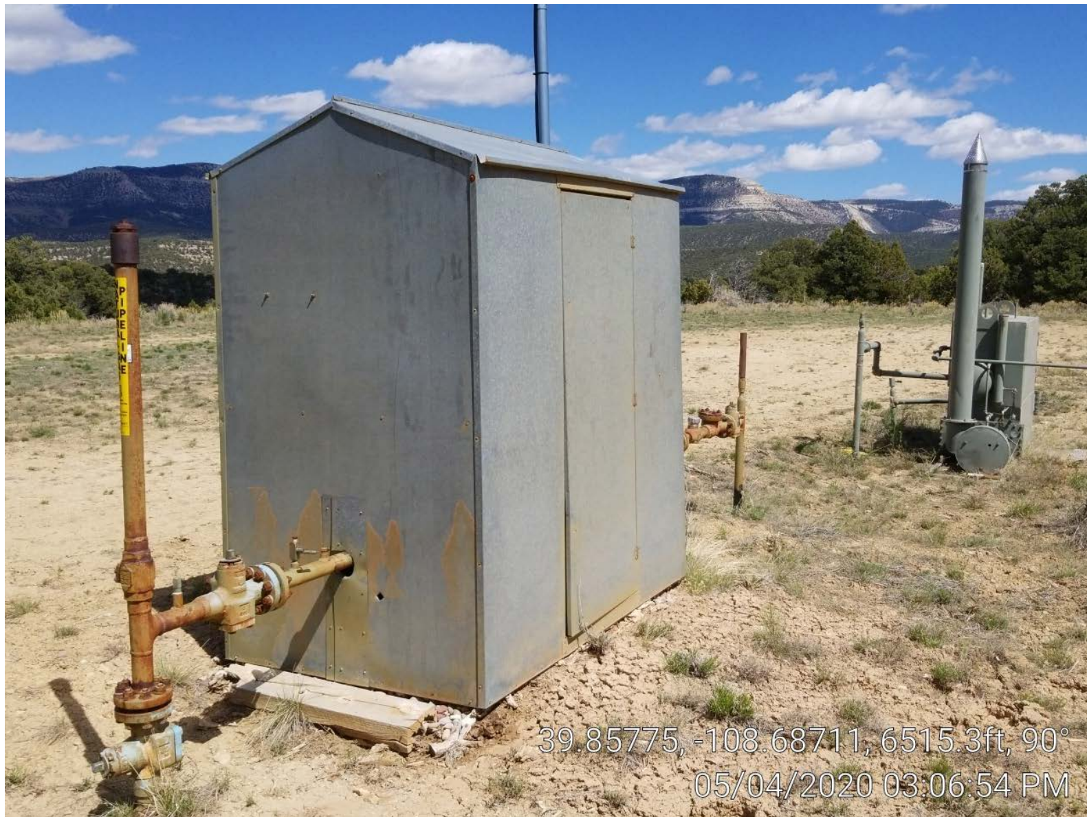
Photo 3. Meter building & separator.
