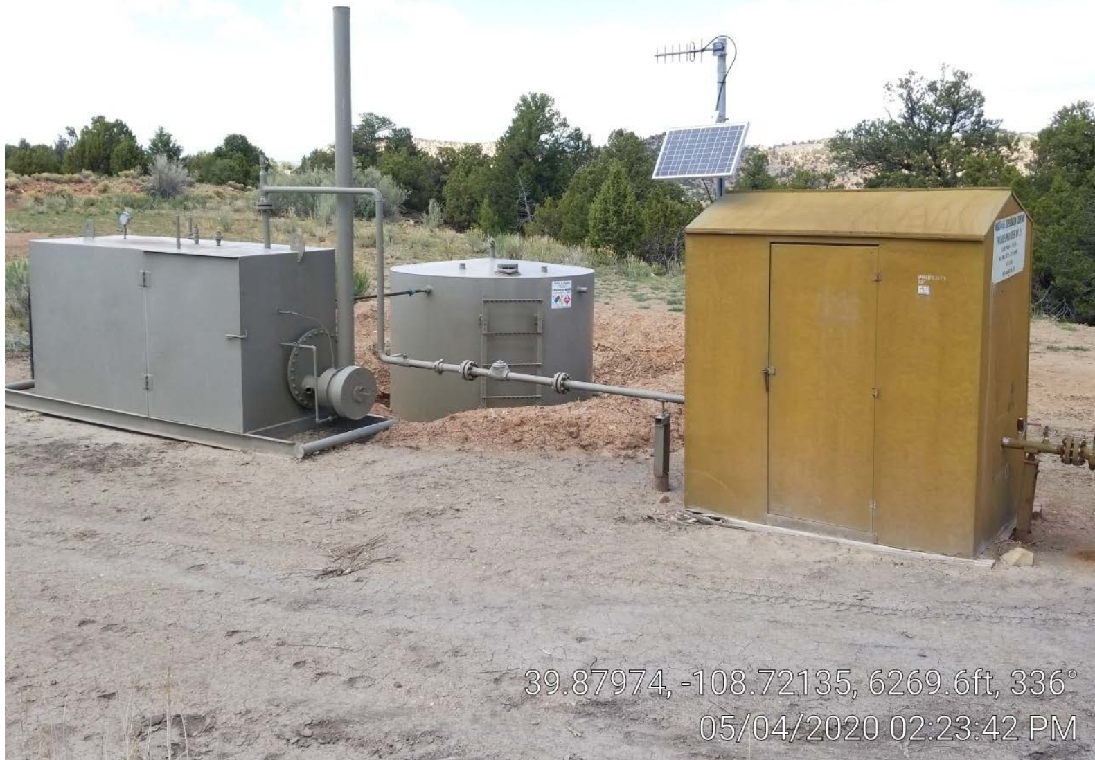
Photo 3. Separator, tank, and meter building.
