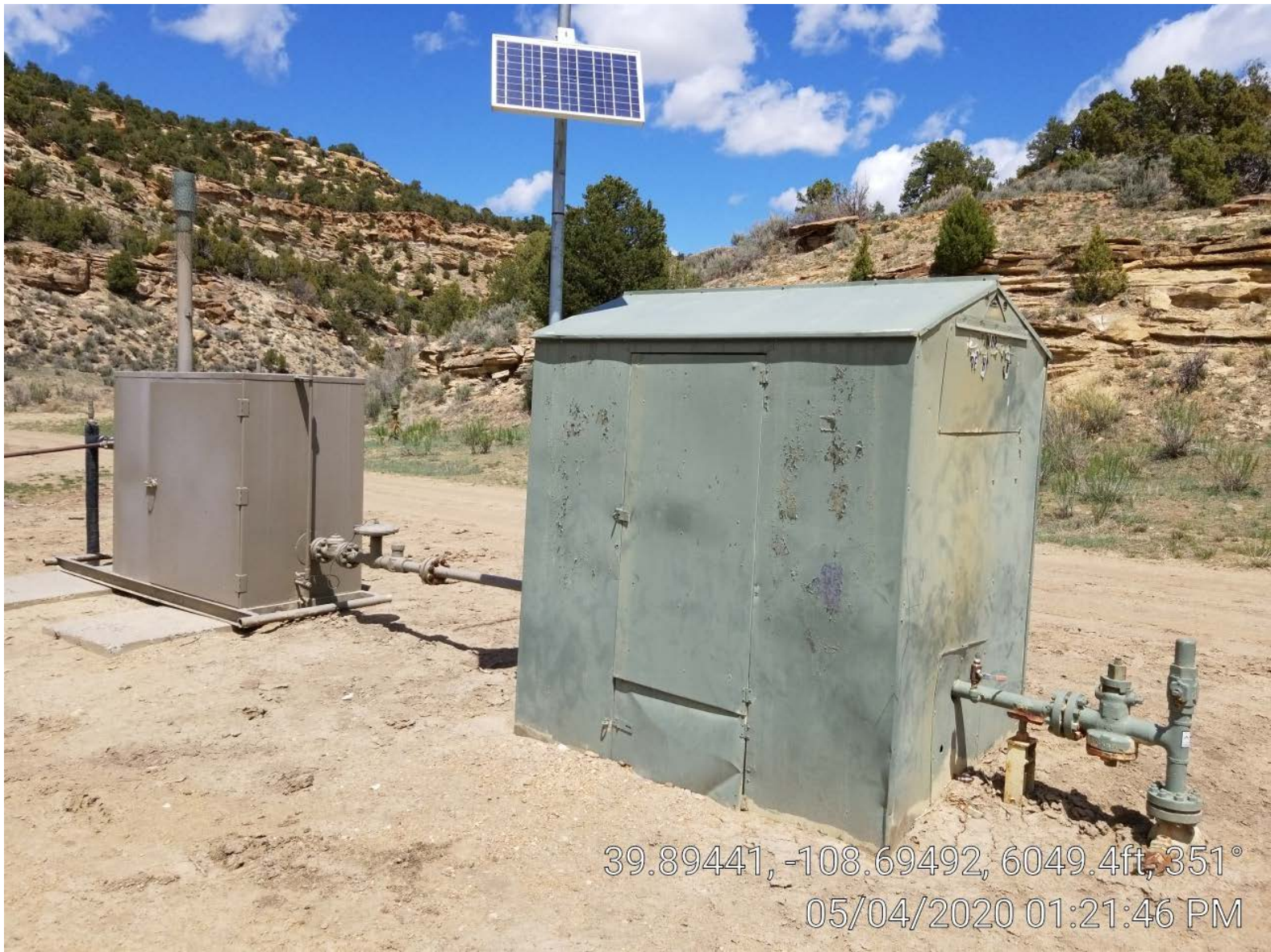
Photo 3. Meter building & separator.
