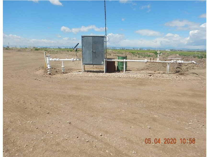
Out of service gas meter run
