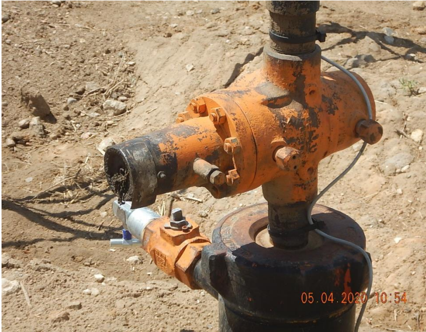
Broken master valve at wellhead.
