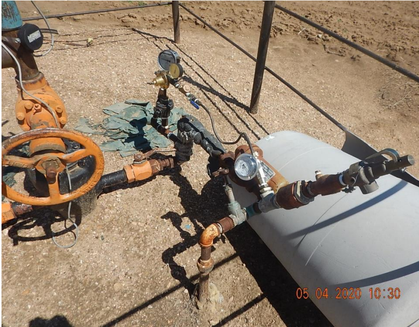
Close up view of domestic tap; Tied into casing, appears to be active (in service).
