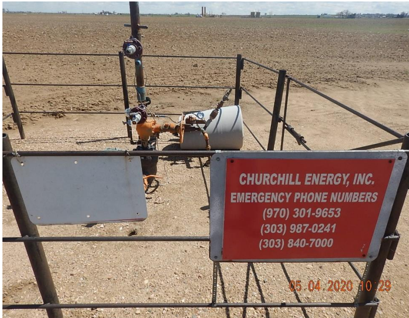
Incomplete signage at wellhead; view North
