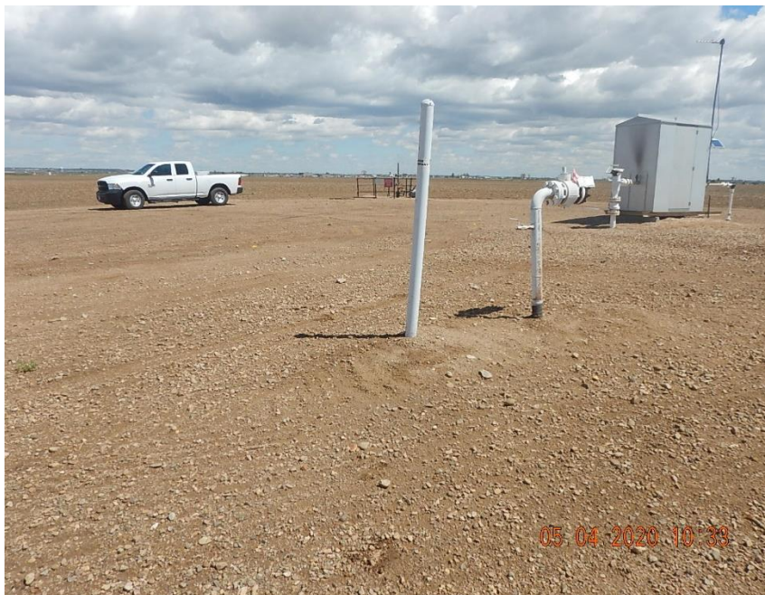
Out of service gas gathering risers in area where production equipment (meter run) has been removed (View NE).
