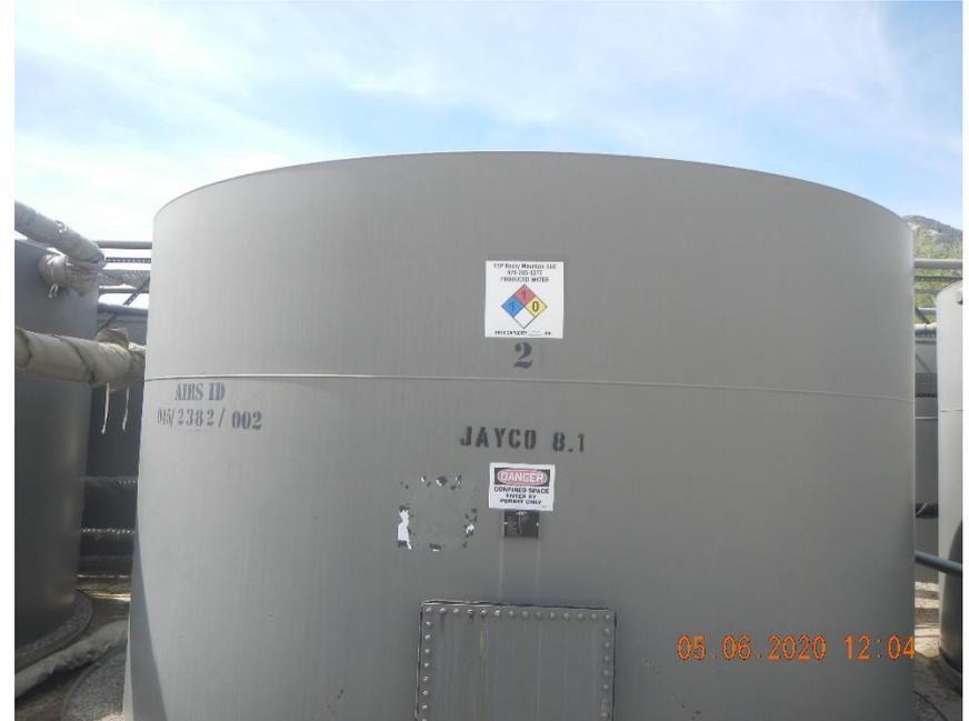
**Tank capacities are faded on tank labels.
