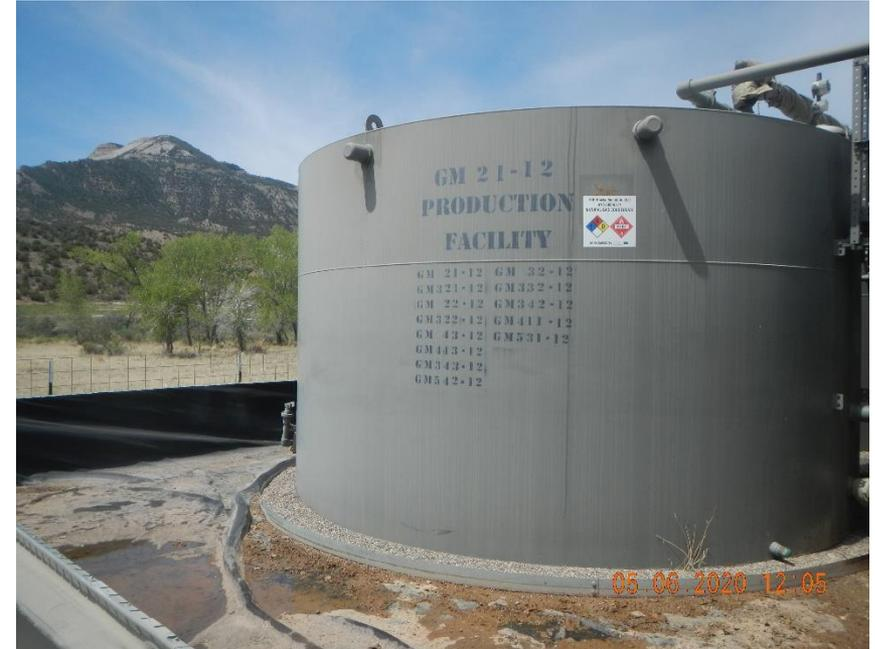
**Tank capacities are faded on tank labels.
