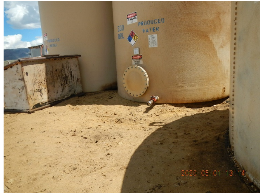
500 bbl produced water tank with load out valve not blind plugged.
