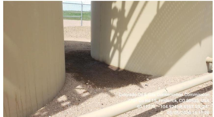
**Photo 13 Stained soil between crude oil tanks**
