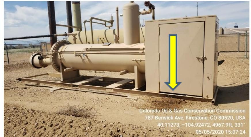
**Photo 9 unused gas meter run**
