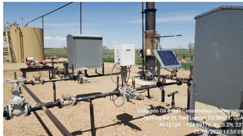
**Photo 9 stained soil under gas meter run**
