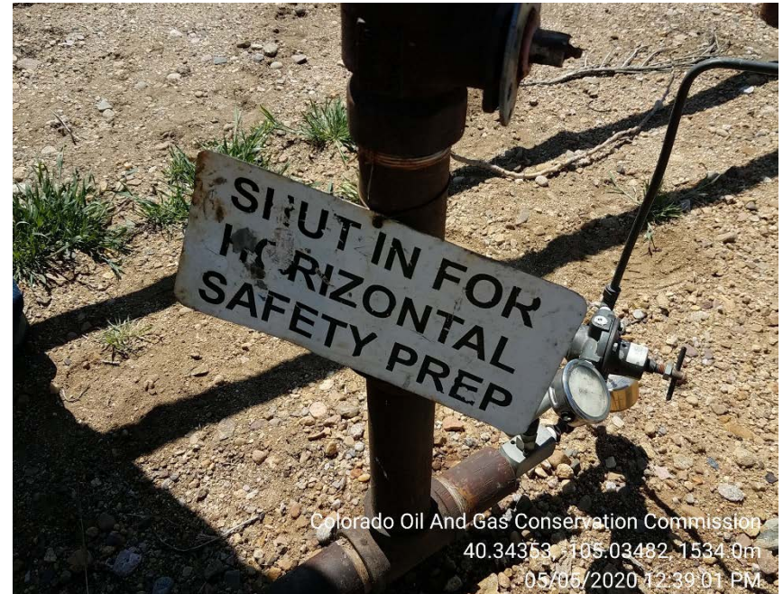
HZ safety prep sign
