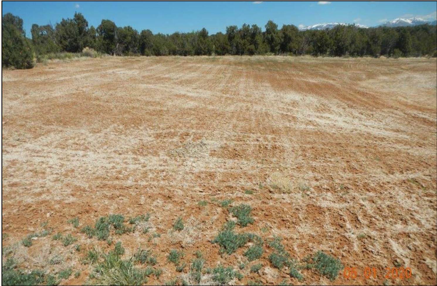
Photo 2. View of the western project area from the southwestern corner facing northward. Cut-slope is recontoured, hydromulched, seeded, and tracked.
