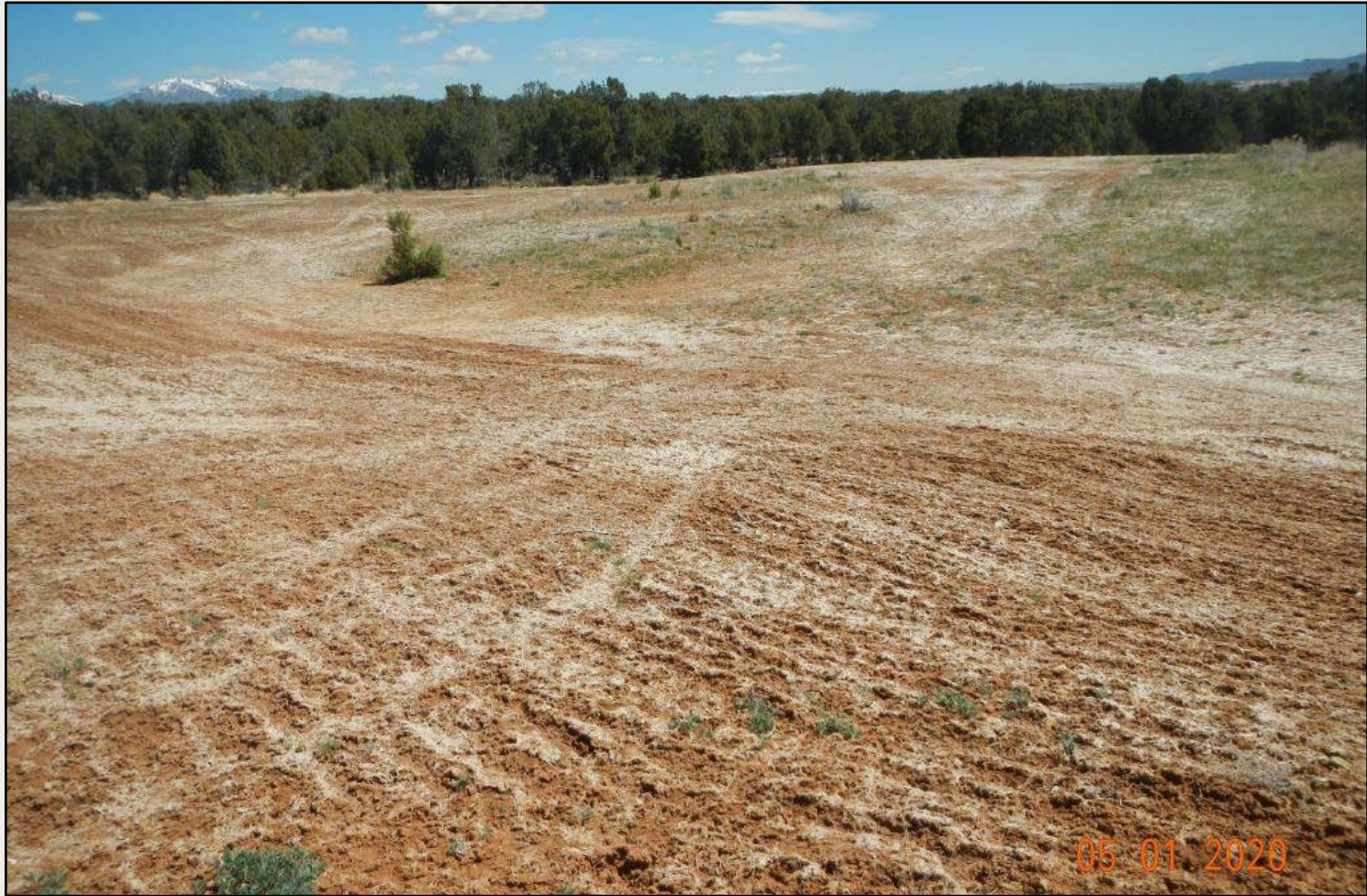
Photo 1. View of the project area from the southwestern corner facing center. The well pad cut and fill slopes are recontoured. A flat portion in the center of the well pad remains flat, as described in the proposed reclamation variance at this location.
