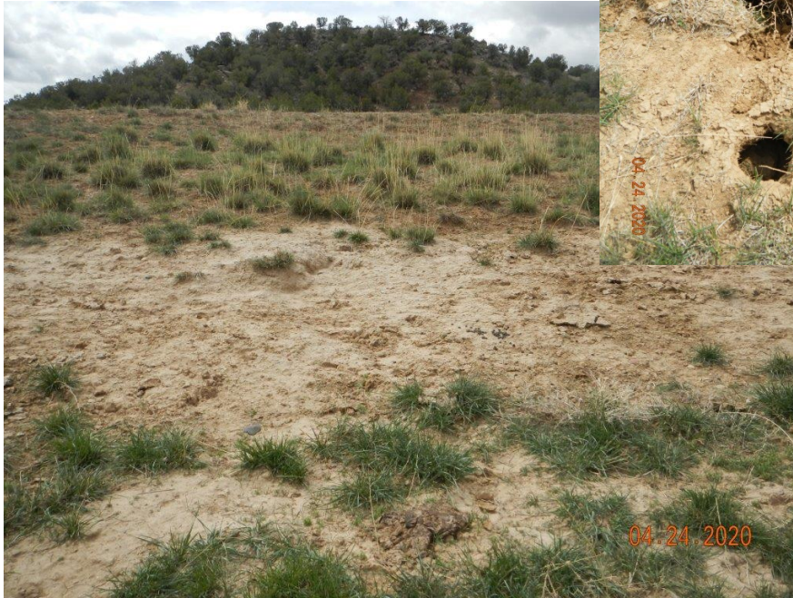
Photo#10: Fill slope and BMPs being de-stabilized, not functioning.
