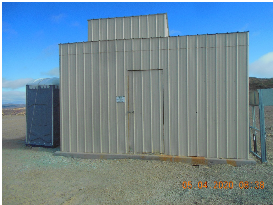
Injection wellhead inside housing.
