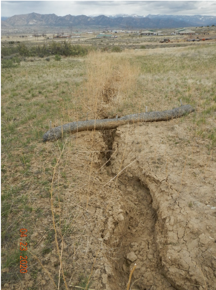
Photo#6: Erosion and non functioning BMP.
