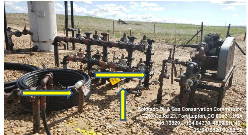
Photo 7 Verical Separator house has been removed
