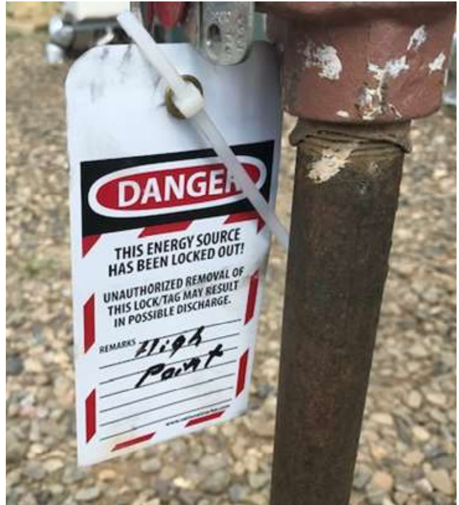
PHOTO 3: THE (2) RISER'S ARE LOW POINT AND HIGH POINT DRAIN'S WHICH ARE IN USE. THE RISER'S WERE LABELED AS TO THE FUNCTION FOR CLARITY.
