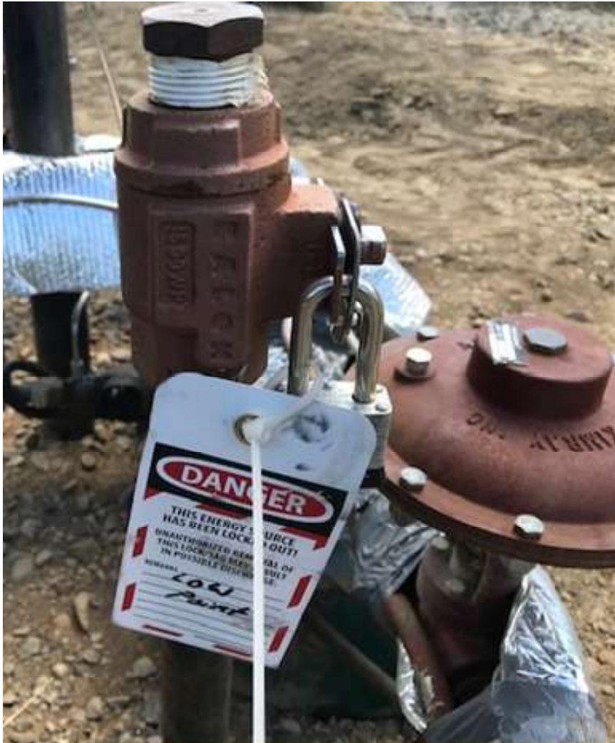
PHOTO 3: THE (2) RISER'S ARE LOW POINT AND HIGH POINT DRAIN'S WHICH ARE IN USE. THE RISER'S WERE LABELED AS TO THE FUNCTION FOR CLARITY.
