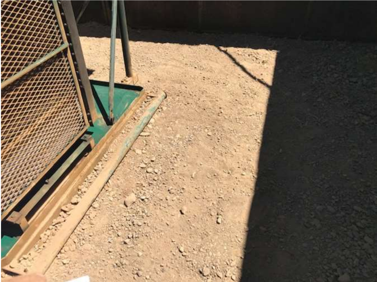
PHOTO 2: THE IMPACTED SOIL/GRAVEL NEAR THE LIQUID RING COMPRESSOR WAS REMOVED AND THE LEAK WAS REPAIRED.
