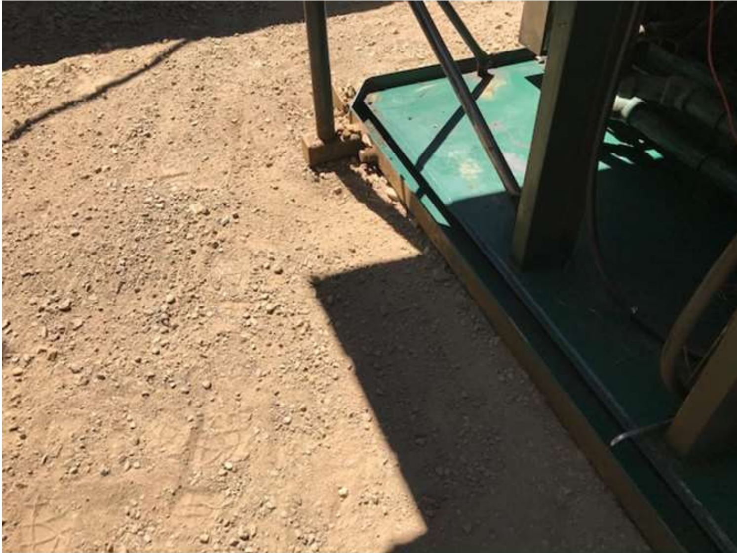
PHOTO 1: MAINTENANCE WAS CONDUCTED TO STOP THE LEAK. THE FLUID ACCUMULATION WAS REMOVED FROM THE LIQUID RING COMPRESSOR SKID AND RESERVOIR. THE IMPACTED SOIL/GRAVEL NEXT TO THE LIQUID RING COMPRESSOR WAS REMOVED FROM THE LOCATION.
