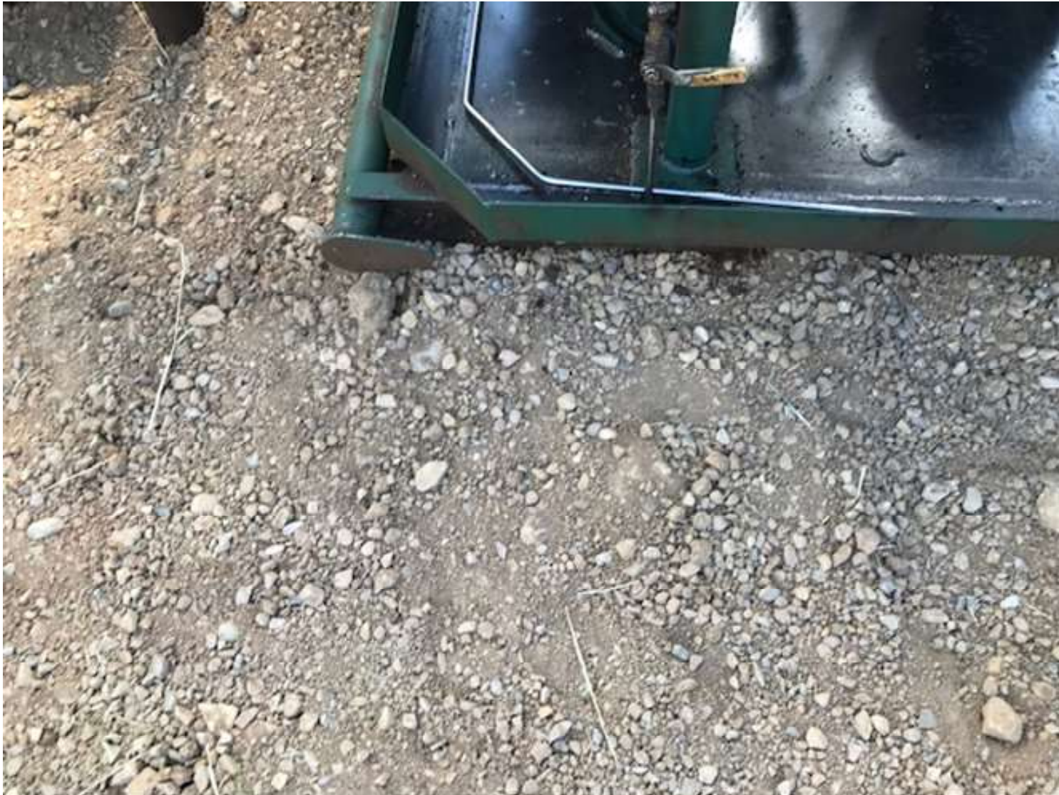
PHOTO 1: MAINTENANCE WAS CONDUCTED TO THE LIQUID RING COMPRESSOR TO STOP THE OIL LEAK. THE IMPACTED SOIL/GRAVEL NEXT TO THE LIQUID RING COMPRESSOR WAS REMOVED FROM THE LOCATION.
