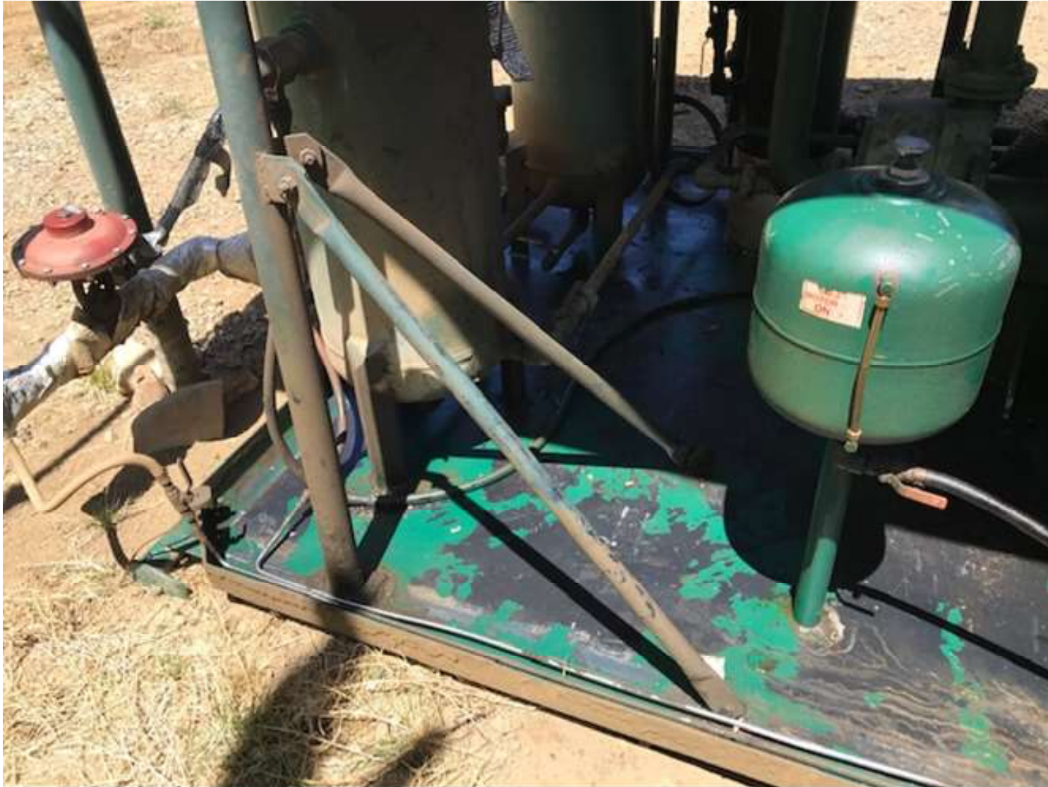
PHOTO 4: MAINTENANCE WAS PREFORMED ON THE LIQUID RING COMPRESSOR. THE FLUID ACCUMULATION WAS REMOVED AND THE SKID WAS CLEANED.
