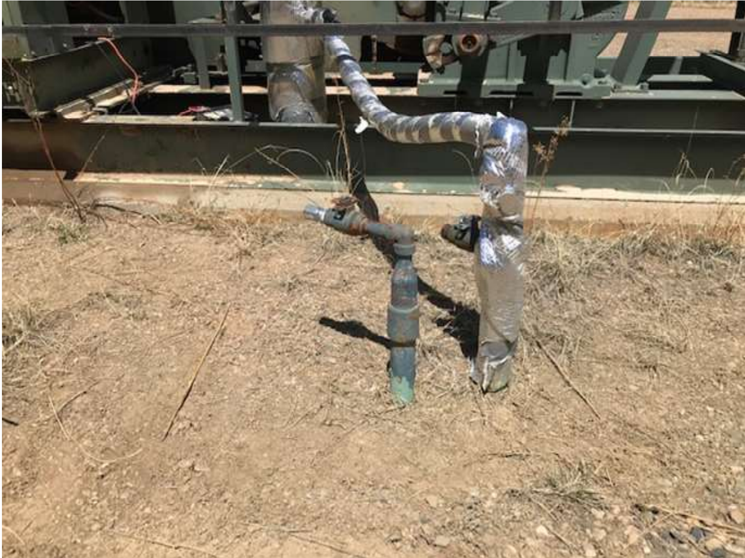
PHOTO 1: THE RISER IS A LOW POINT DRAIN AND IS IN USE. THE RISER WAS LABELED AS TO THE FUNCTION FOR CLARITY.
