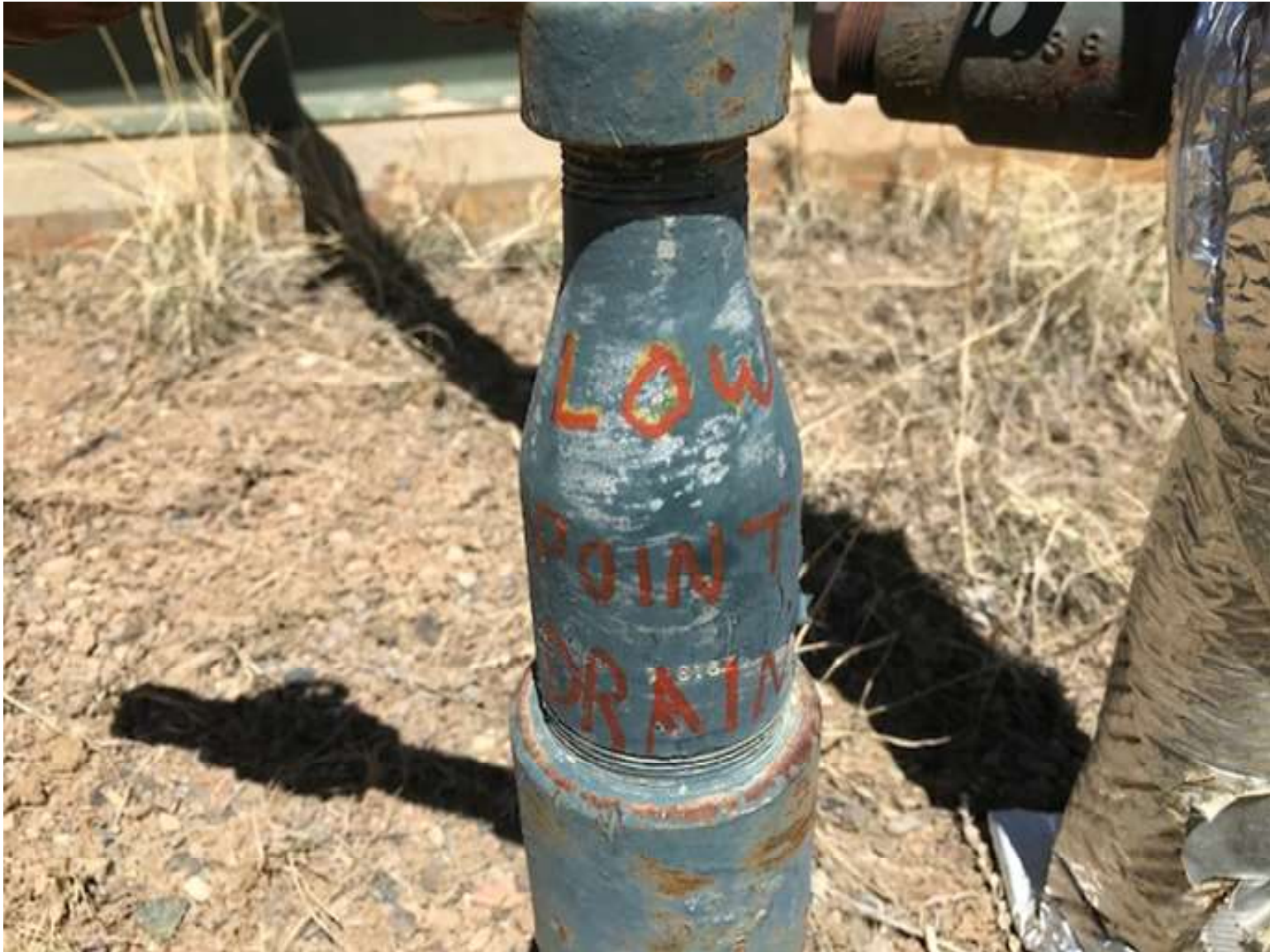
PHOTO 2: THE RISER IS A LOW POINT DRAIN AND IS IN USE. THE RISER WAS LABELED AS TO THE FUNCTION FOR CLARITY.
