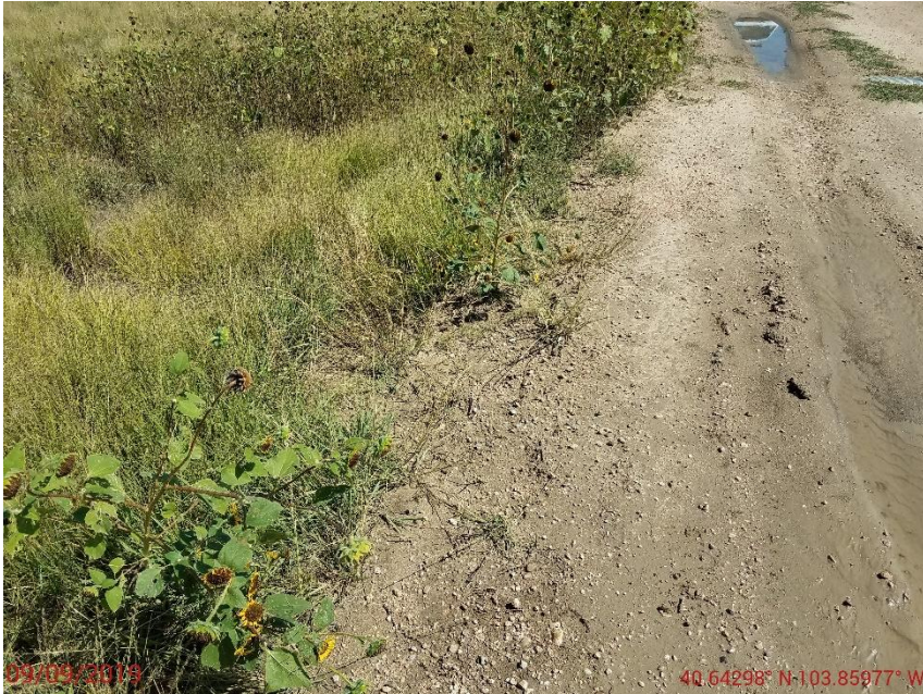
Photo 3: Photo shows areas where stormwater from the access road is discharging onto the adjacent lands. Sediment deposition evident.
