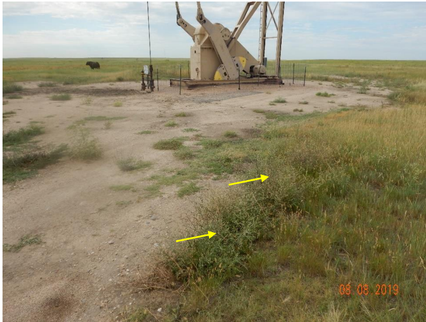
Photo 1: Photo taken from north end of the location, facing south. Photo provides an overview of the location. Photo shows Diffuse Knapweed (Plants with white flowers in photo) remains established on the location/access road. Operator has failed to conduct sufficient ongoing noxious weed management on the location.
