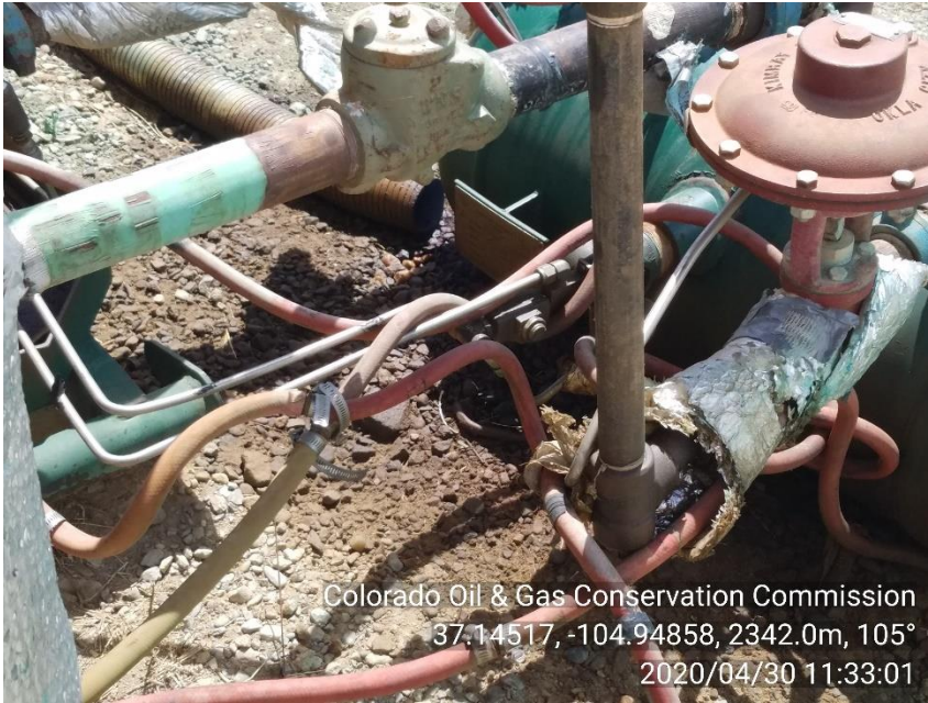
PHOTO 5: IMPACTED SOIL NEAR AND AROUND COMPRESSOR SKID. Conduct maintenance on equipment, cleanup stained material and review self inspection processes. 5-7-20.
