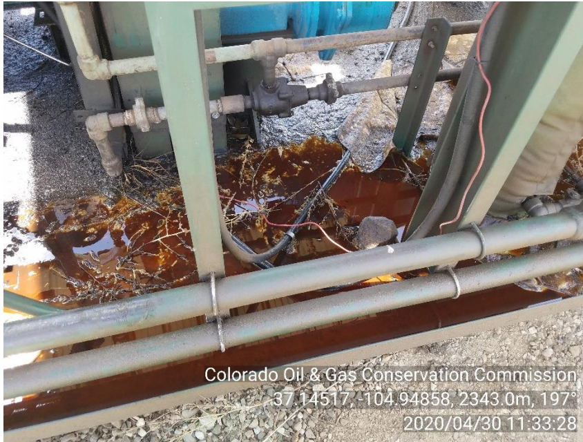
PHOTO 3: STANDING OIL IN COMPRESSOR SKID. APPEARS THAT ENGINE OIL IS BEING DRAINED INTO SKID. Comply with general provisions of the oil and gas act for wildlife protection. CA DATE 5-7-20.
