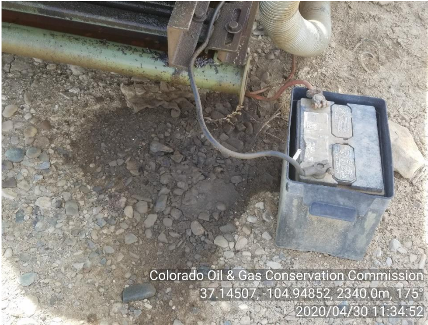
PHOTO 7: IMPACTED SOIL NEAR AND AROUND PRIME MOVER ENGINE SKID. Conduct maintenance on equipment, cleanup stained material and review self inspection processes. 5-7-20.
