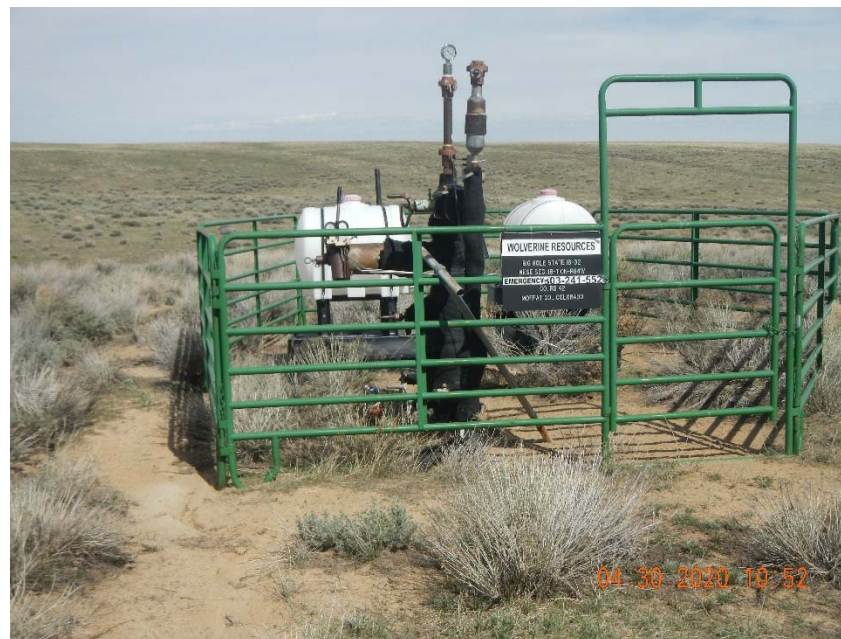
Photo 2. Wellhead with hissing sound coming from leak.
